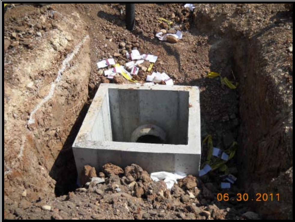
Underground Concrete Storm Box
