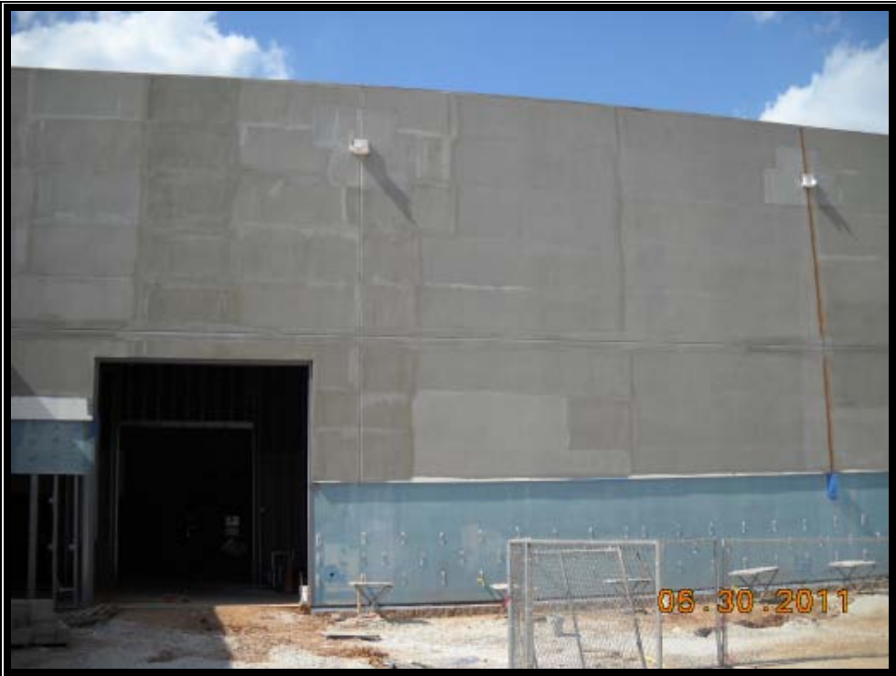
Installation of EIFS on South Side of Building
