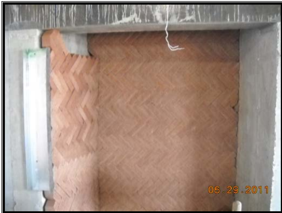
Installation of Brick Fireplace in Multipurpose Room E103
