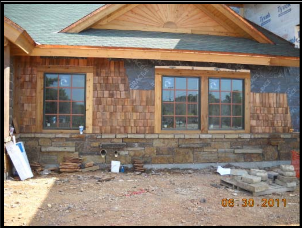
Installation of Cedar Shakes on North Elevation
