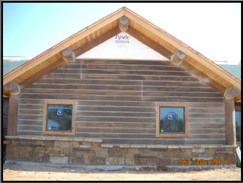
Installation of Fiberglass Siding and Fiberglass Timbers
