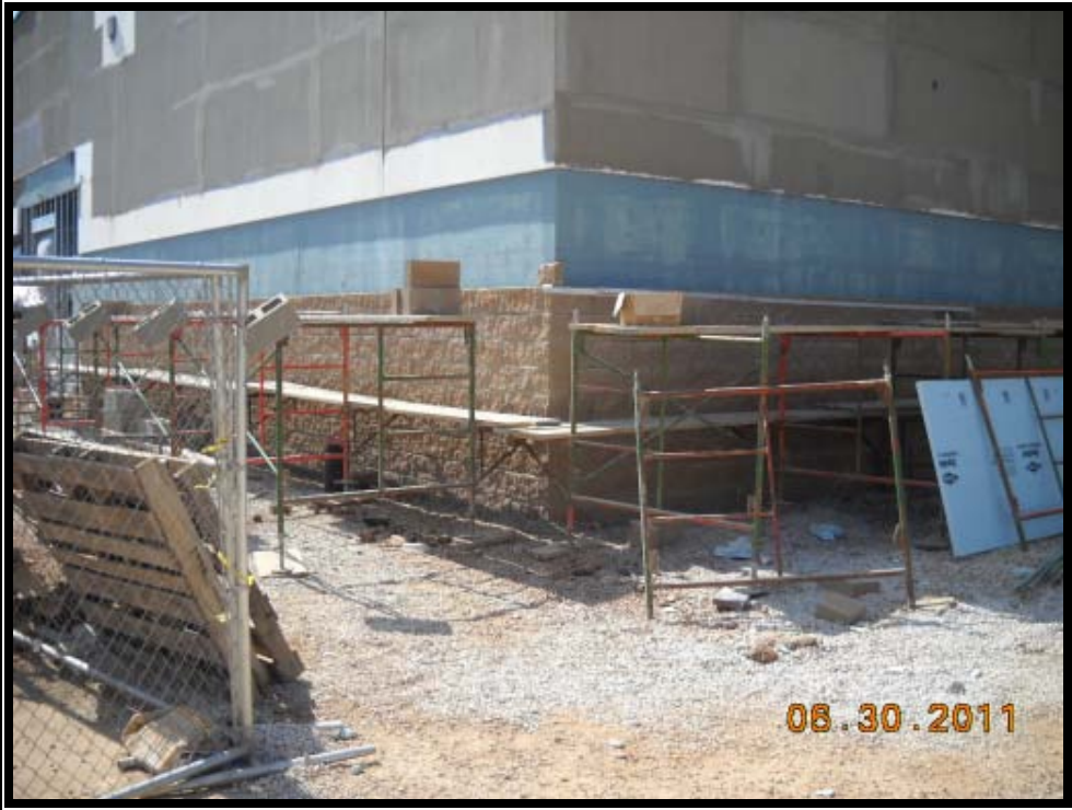
Installation of Exterior Concrete Masonry Units on South Side of Building
