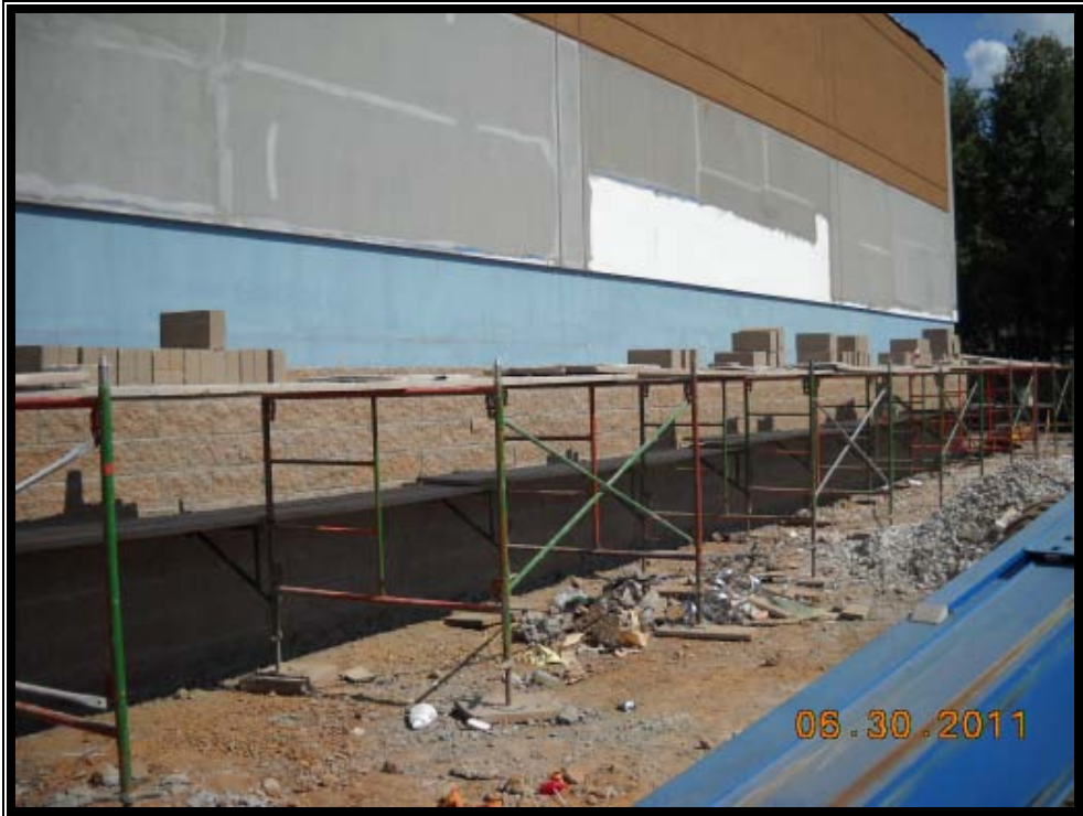
Installation of Exterior Concrete Masonry Units on West Side of Building
