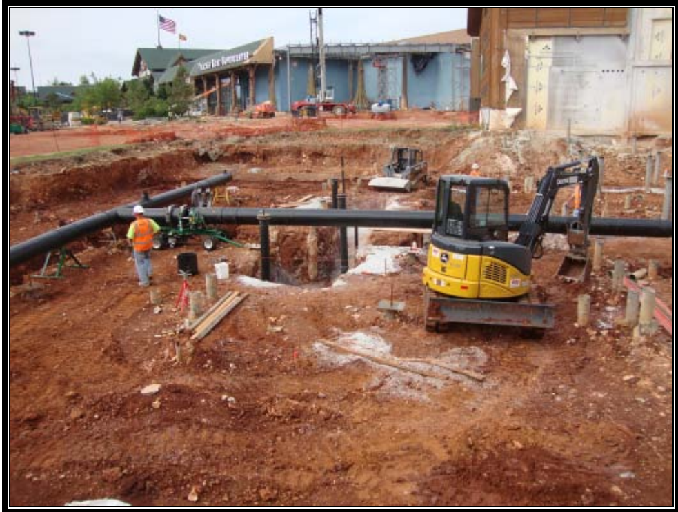
Underground LSS Pipe Installation
