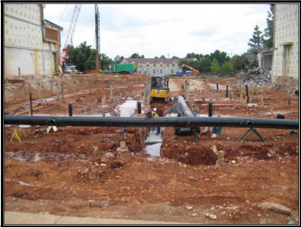
Underground LSS Pipe Installation
