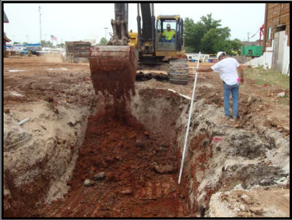
Excavation of the Pit Continued
