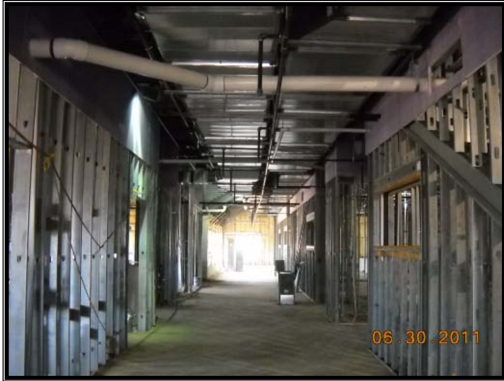
Installation of Conduit, Sprinkler Systems & HVAC in Corridor
