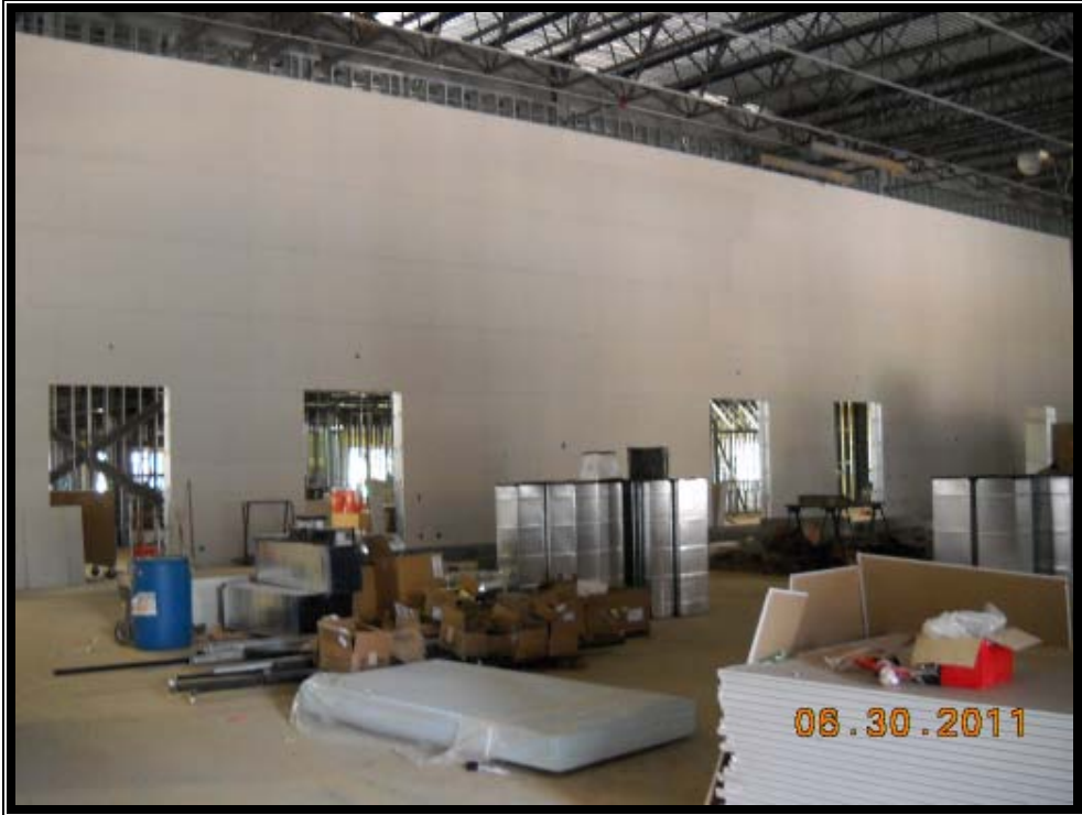
Installation of Gypsum Wall Board in the Expo Hall
