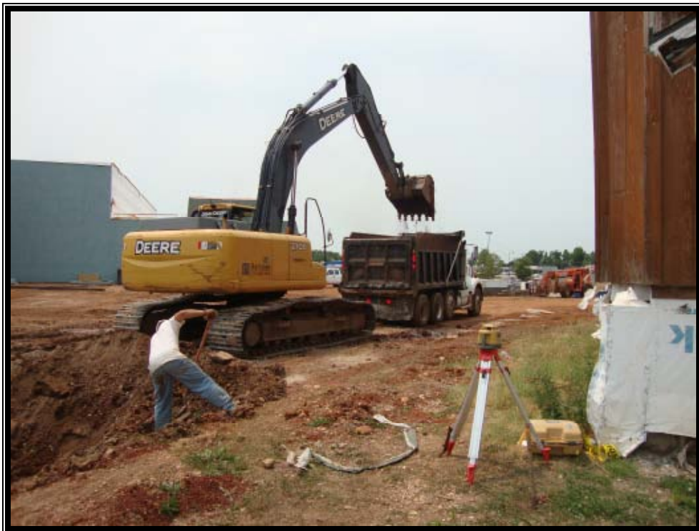
Excavation of the Pit Continued
