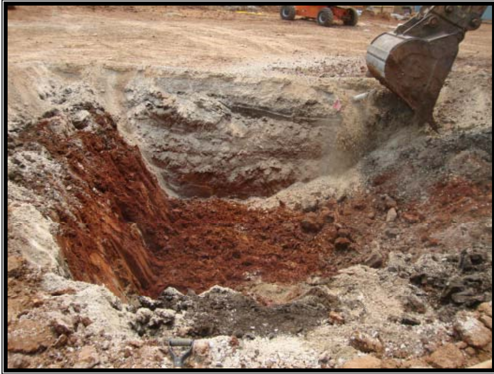
Beginning of Excavation for the Pit
