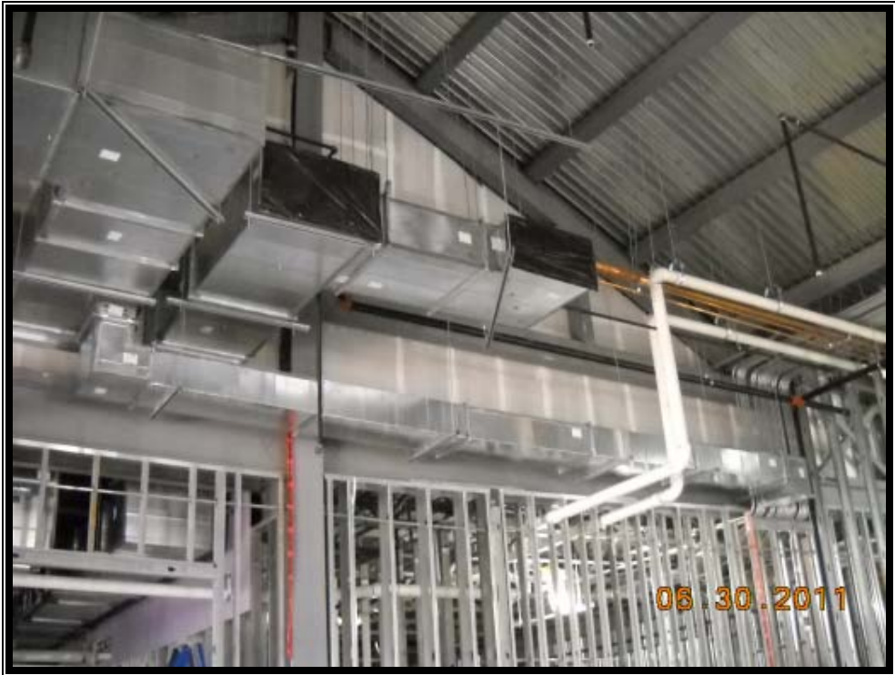
Installation of Conduit, Sprinkler Systems & HVAC in Lobby E137
