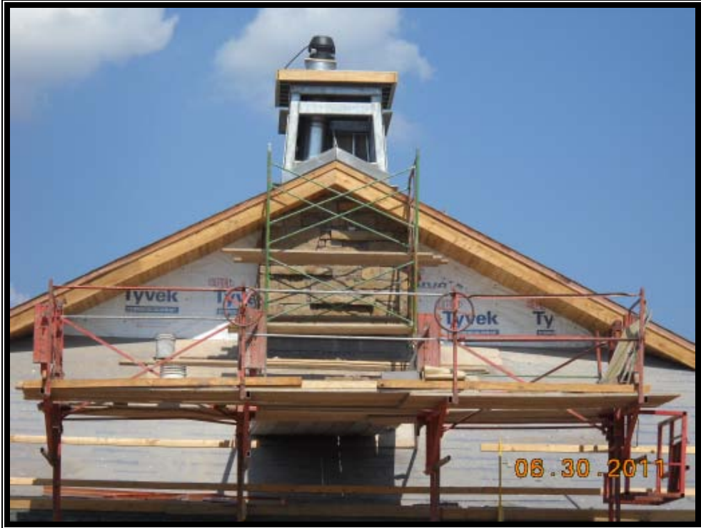
Rock Installed on Chimney
