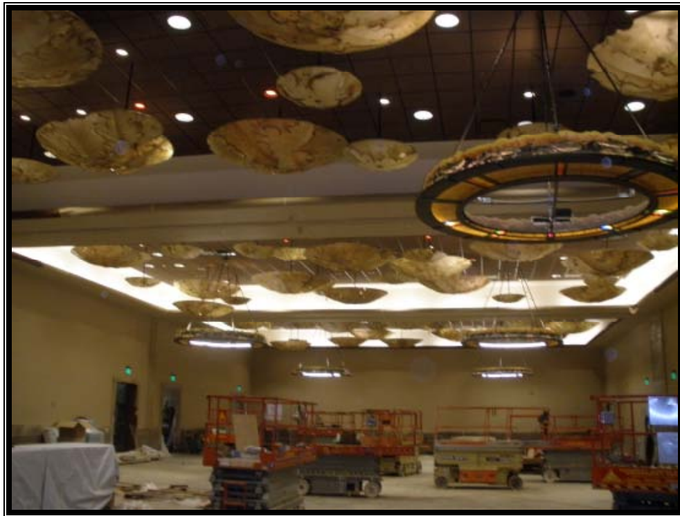
Installation of Rawhide Domes & OFCI Chandeliers in Expo Halls
