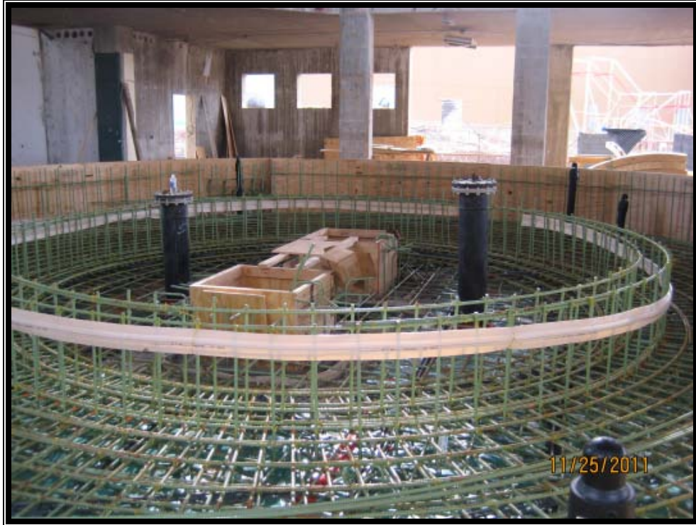
Stingray Tank Foundation Rebar
