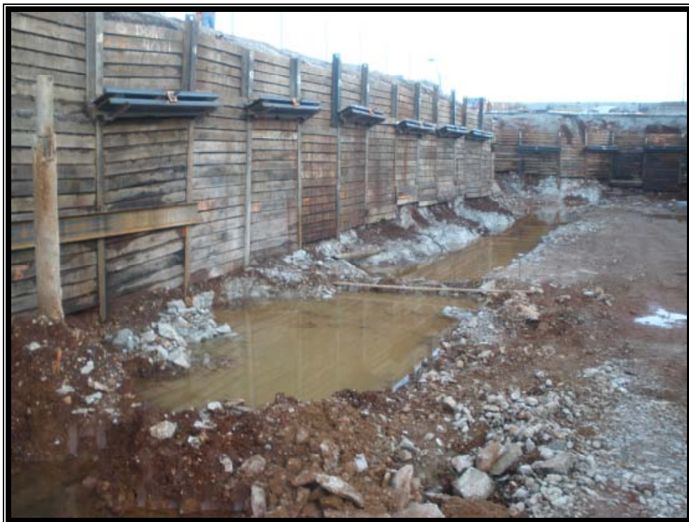
Snapshot of Connector Excavation
