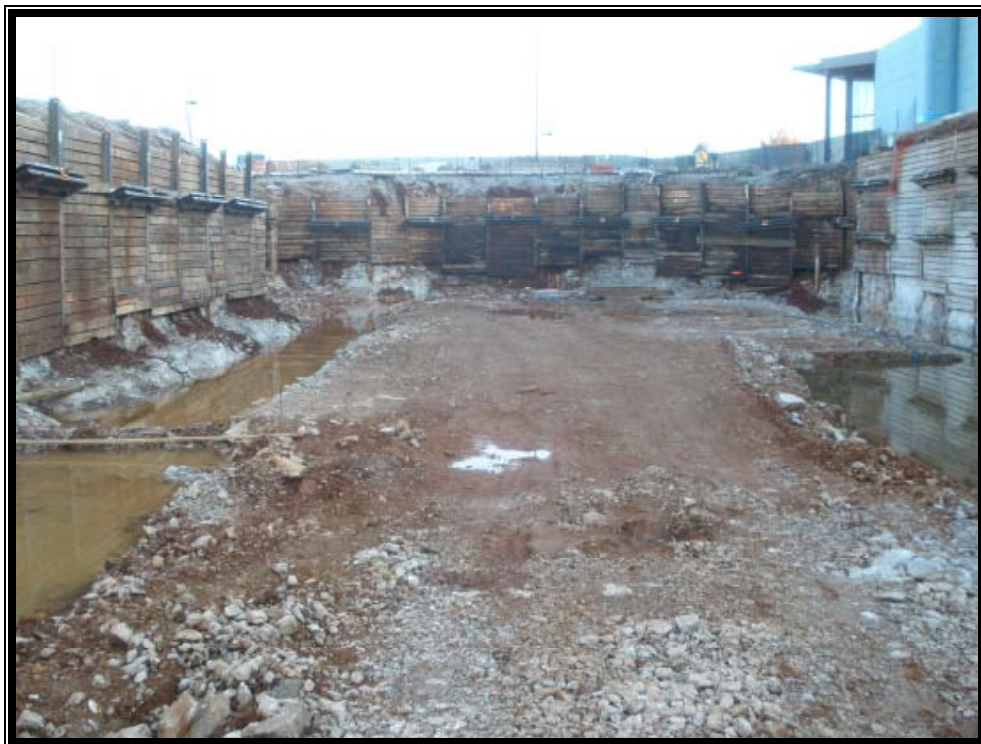
Snapshot of Connector Excavation
