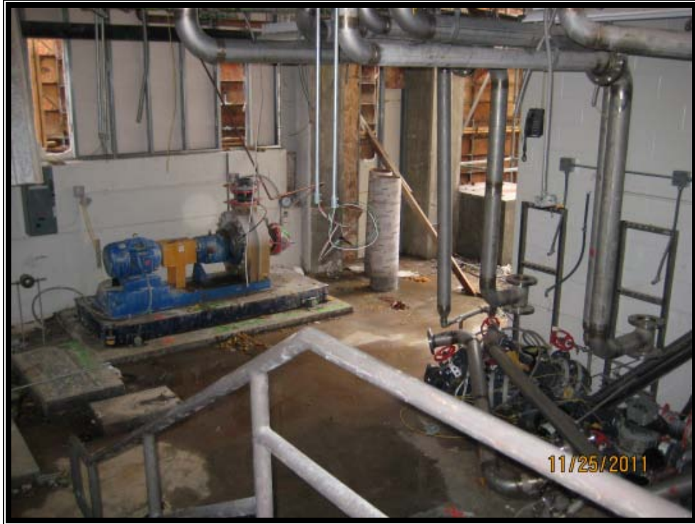
Mechanical Room Demolition
