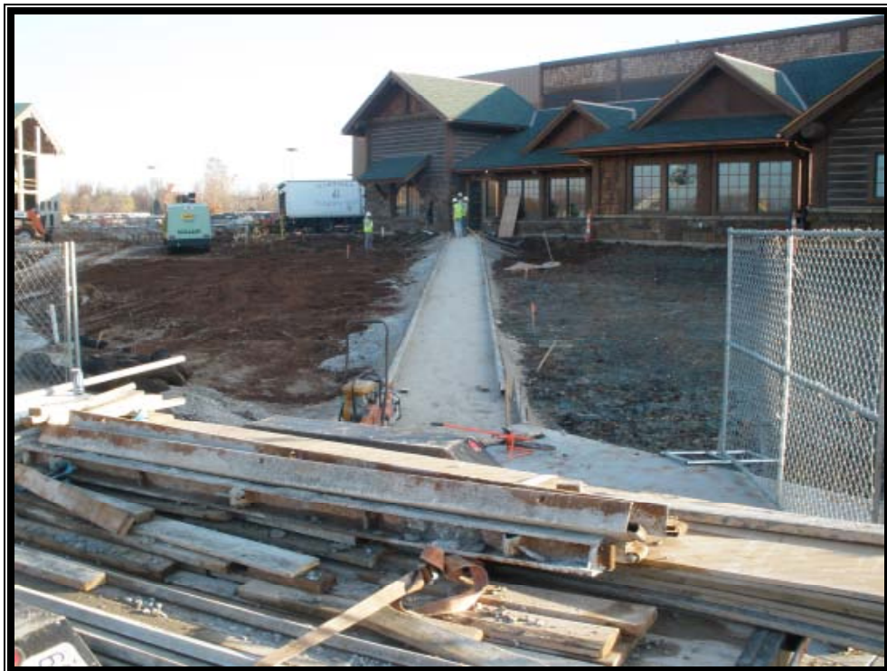
Installation of Sidewalk at Expo/CEC
