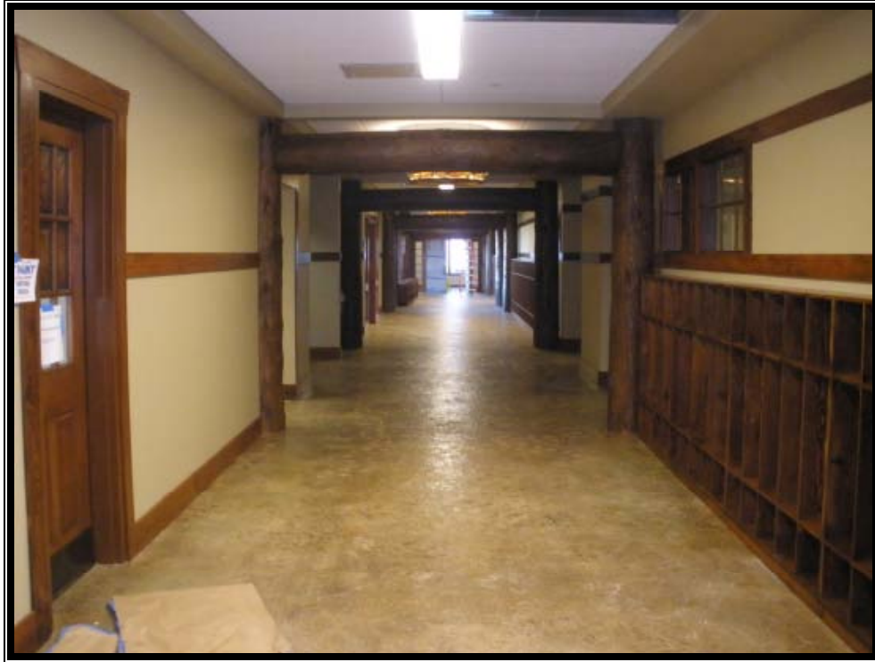
Snapshot of Corridor E104 with Floor Protection Removed
