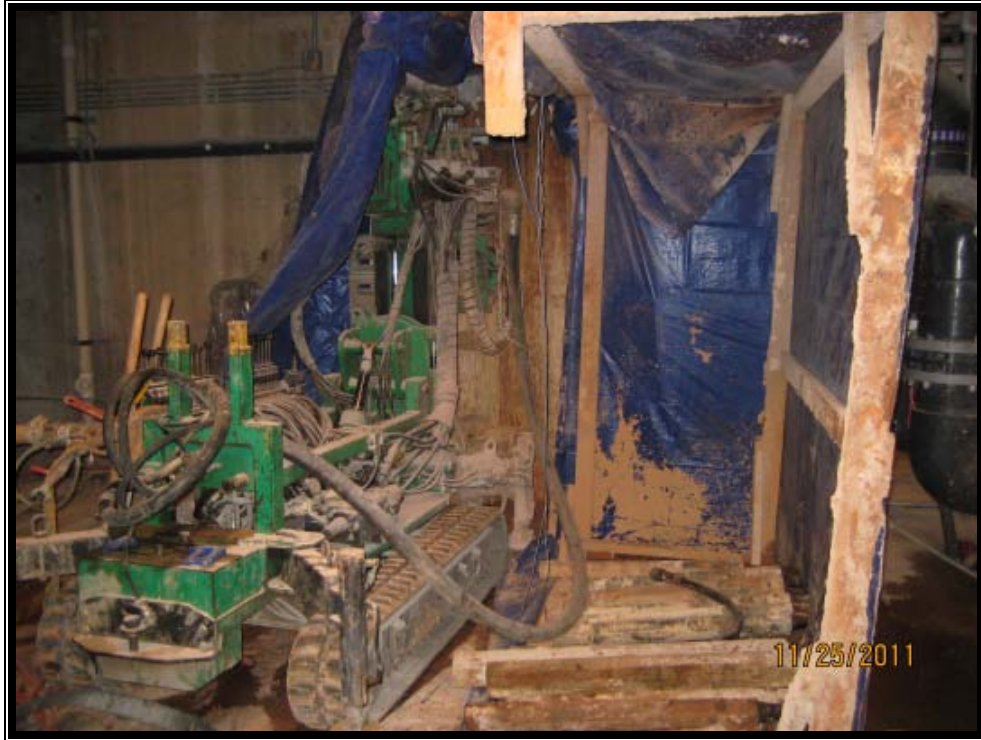
Basement Macro-Pile Installation
