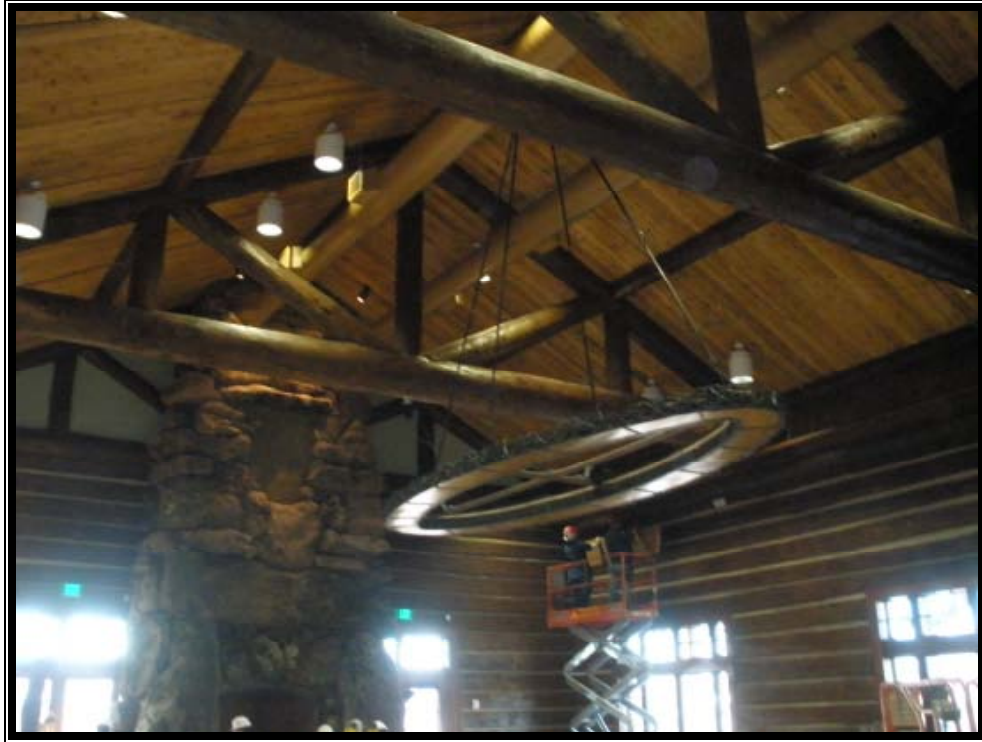
Installation of OFCI Chandelier in Multipurpose Room E103
