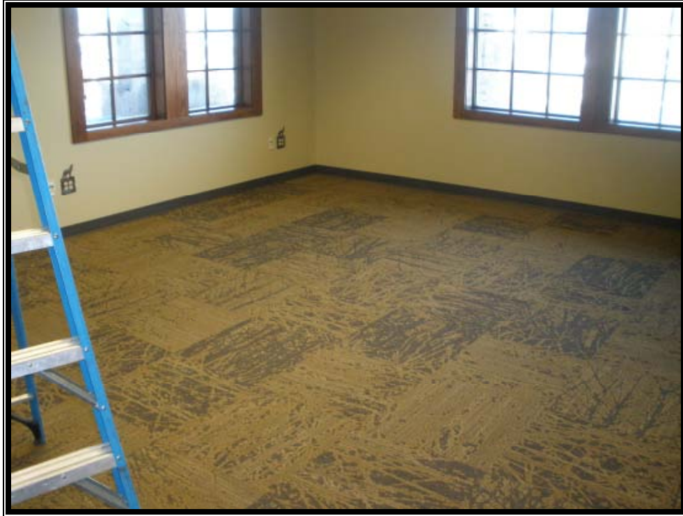
Snapshot of Office E105 with Floor Protection Removed
