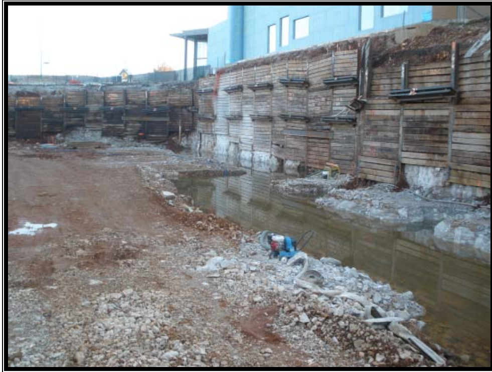
Snapshot of the Connector Excavation
