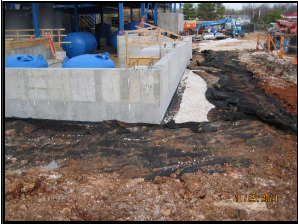
Foundation Wall Backfill
