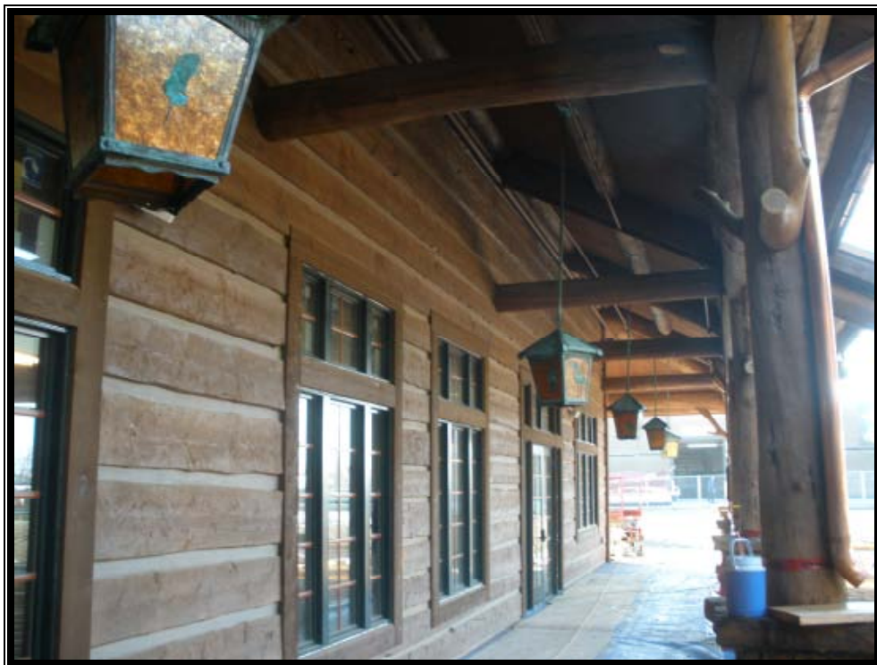
Installation of OFCI Lanterns at Covered Porch
