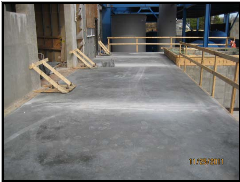
Elevated Floor Slab Completion
