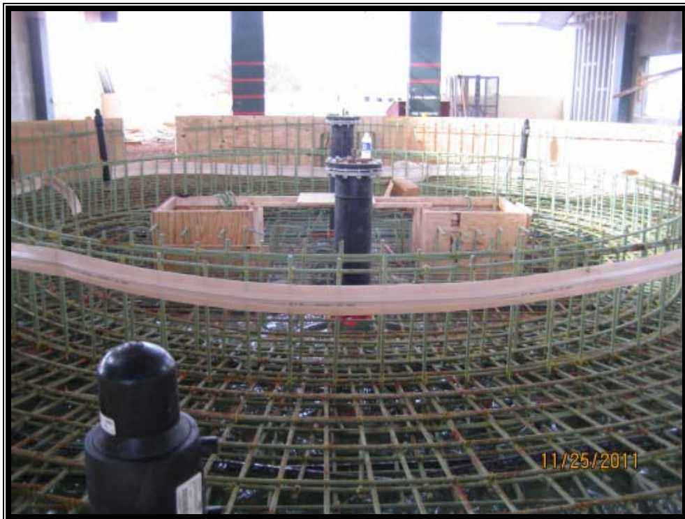
Stringray Tank Foundation Rebar
