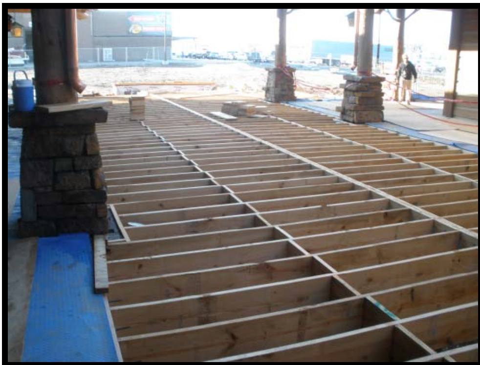
Installation of Wood Deck Framing
