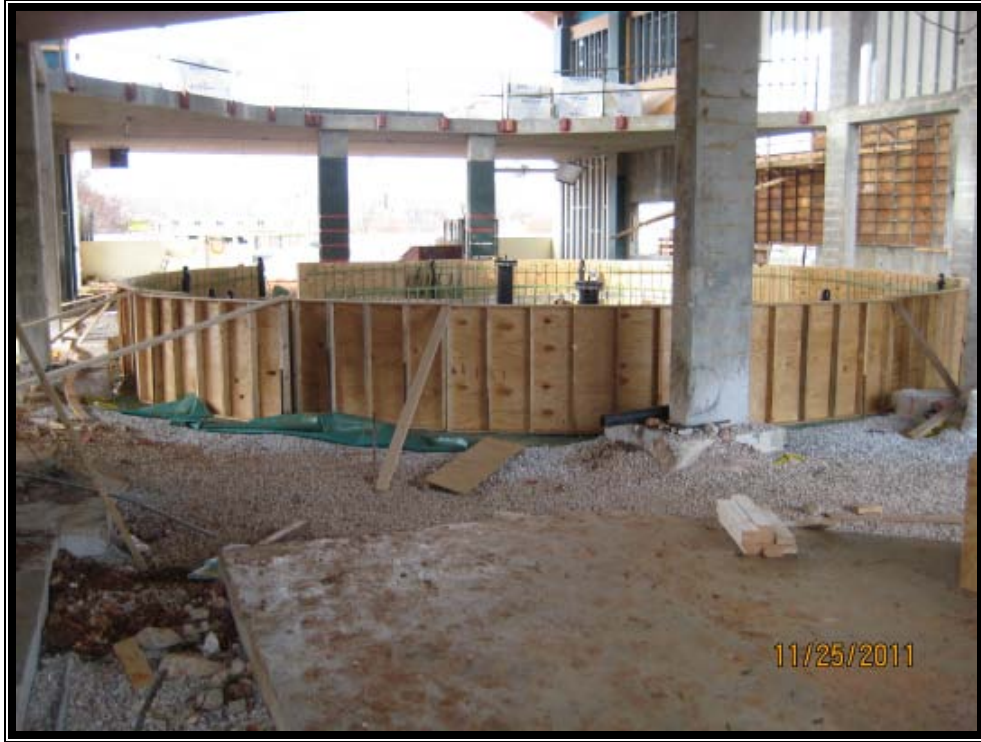
Stingray Tank Foundation Forms
