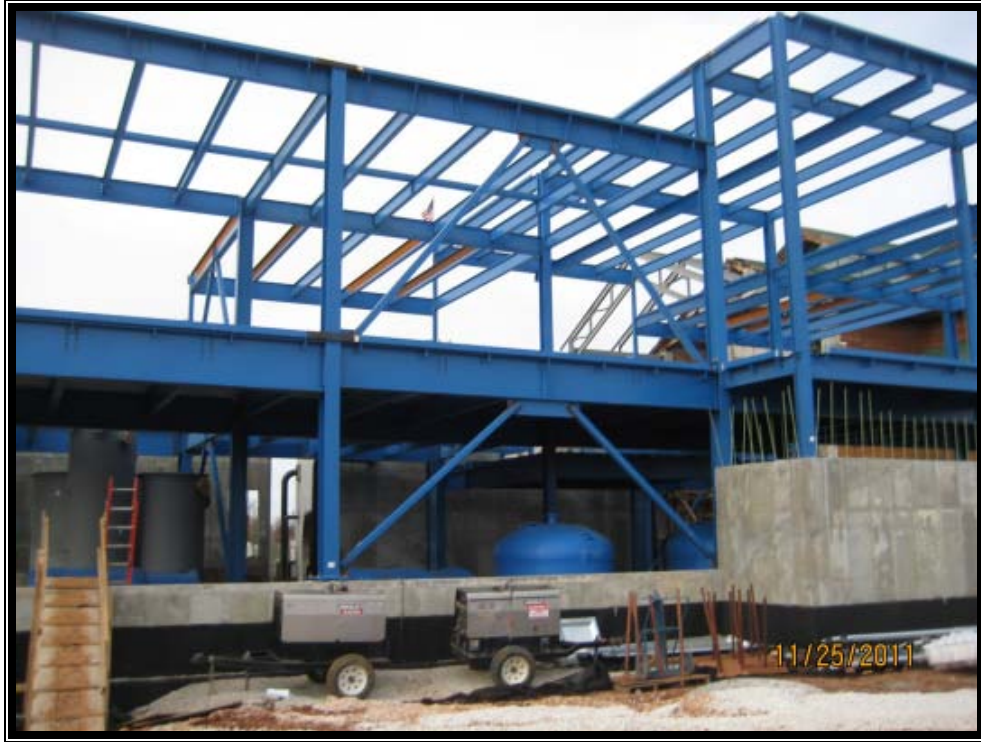
Back of House Structural Steel
