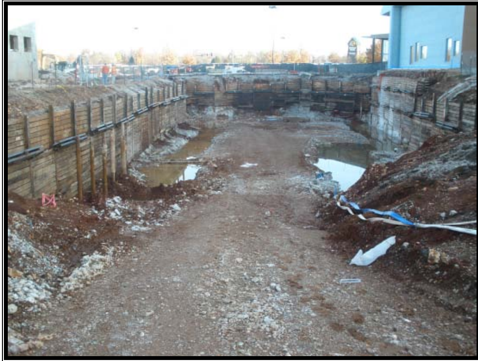
Snapshot of the Connector Excavation
