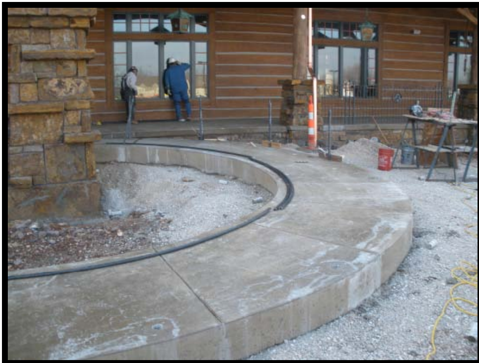
Installation of Handicap Ramp Railing
