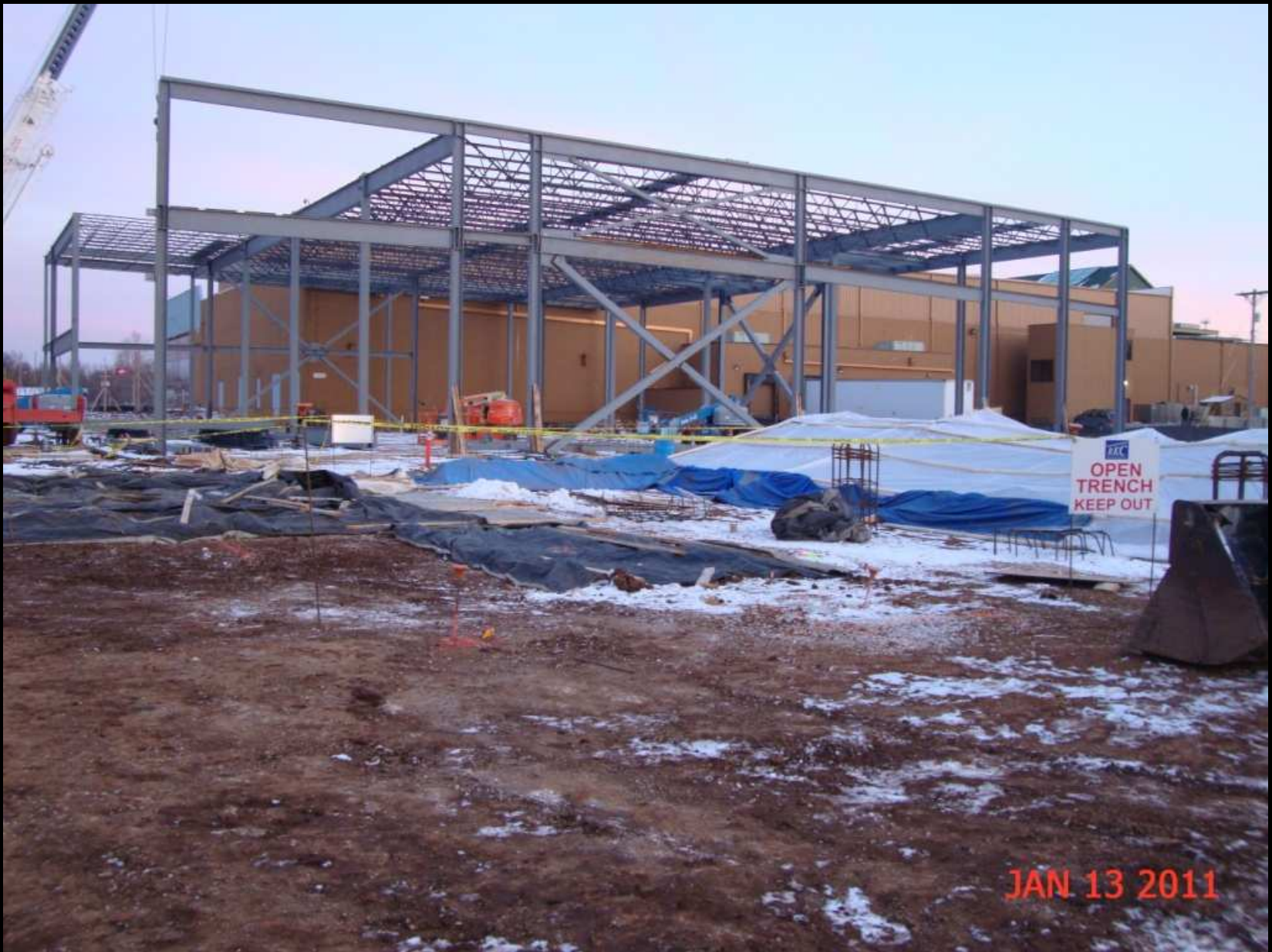
Concrete Foundations Protection
