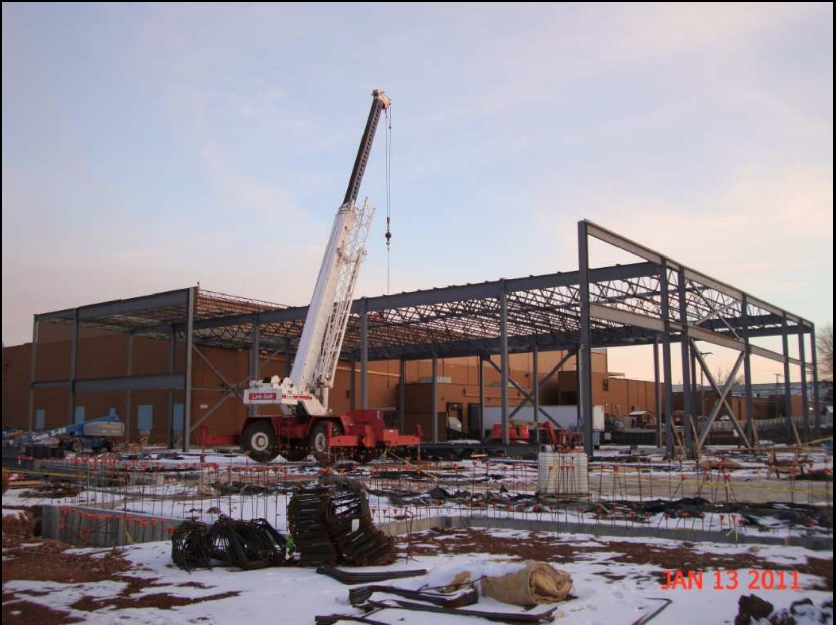
Steel Erection
