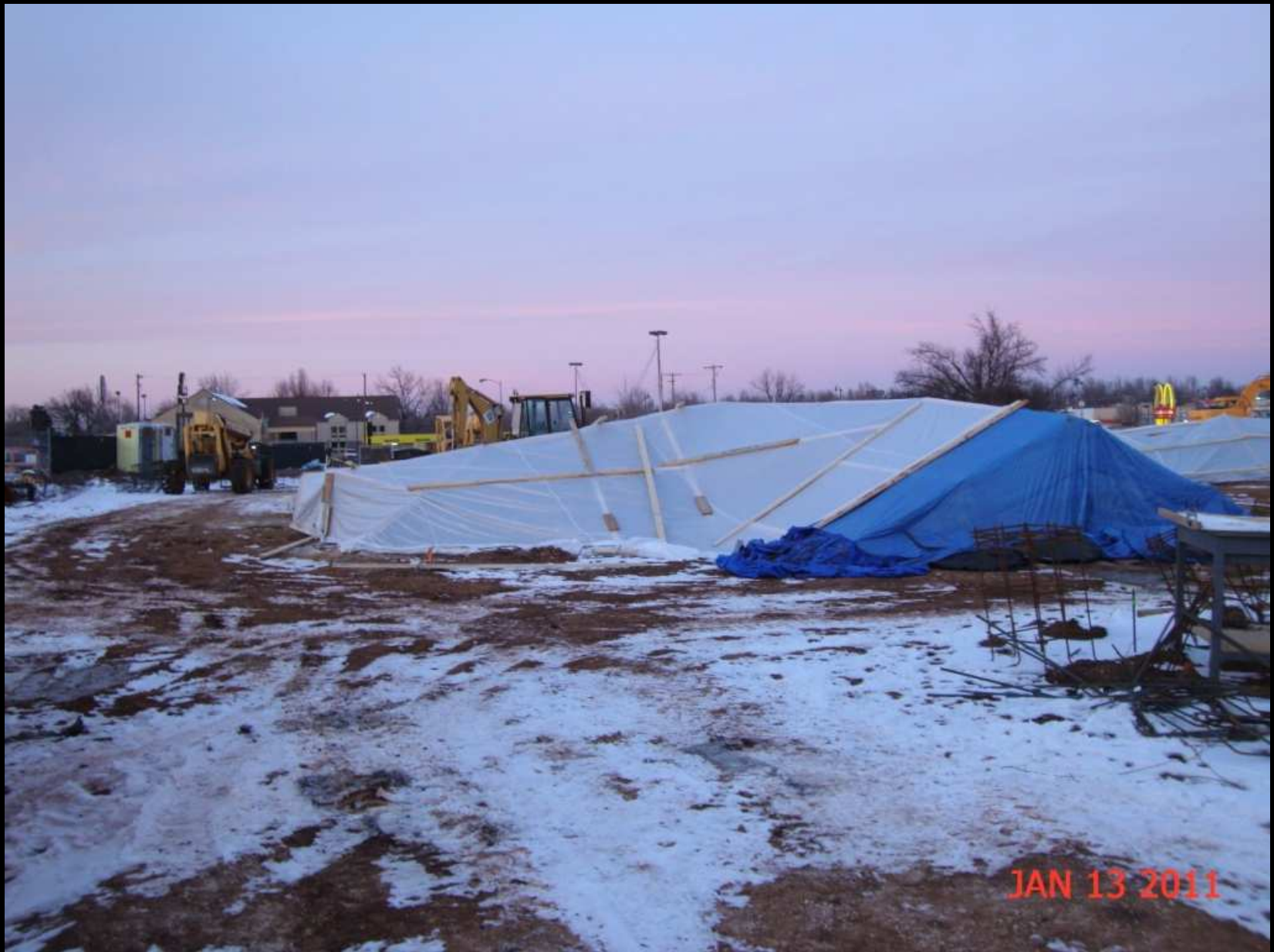
Concrete Foundations Protection
