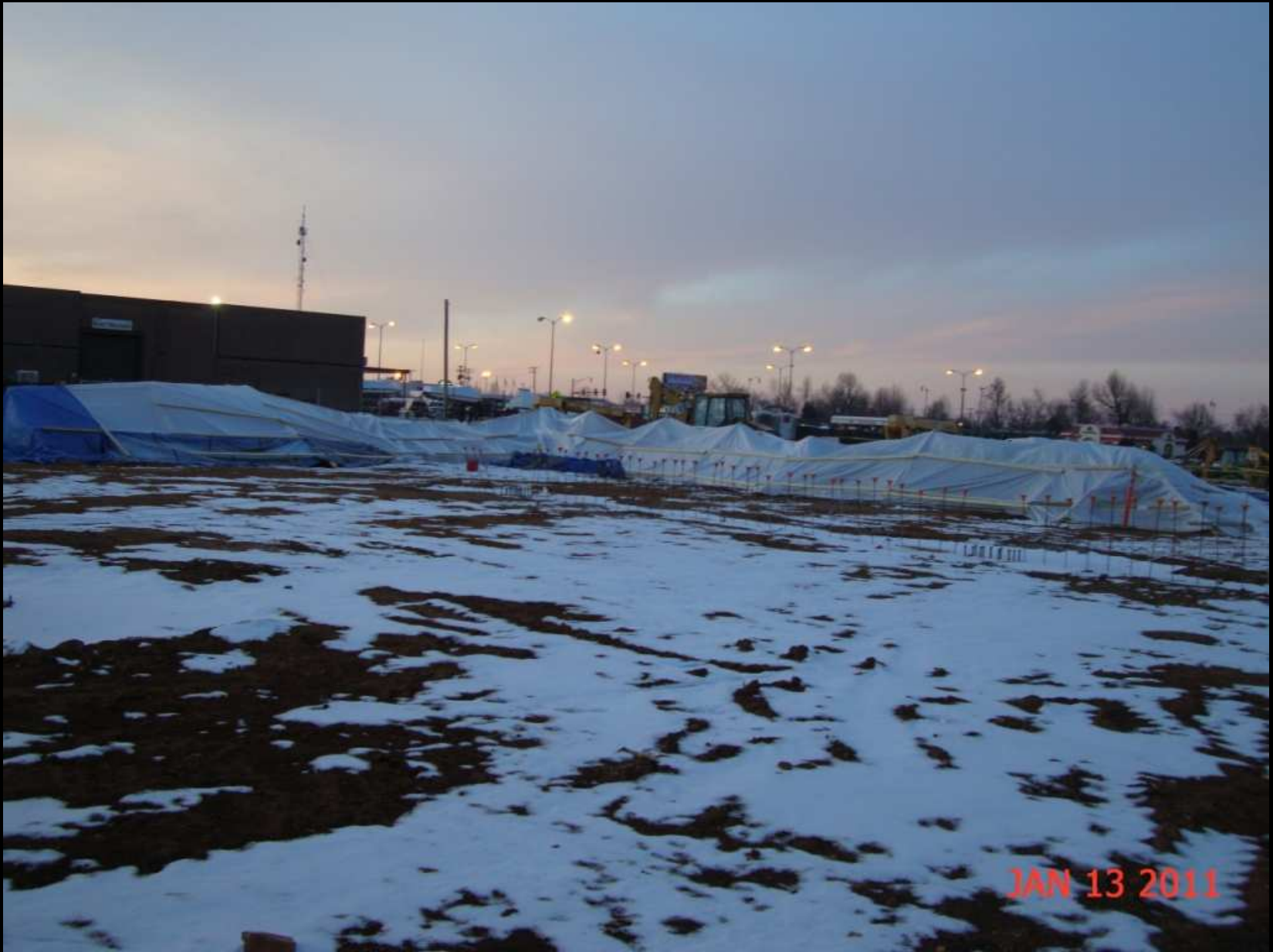
Concrete Foundations Protection
