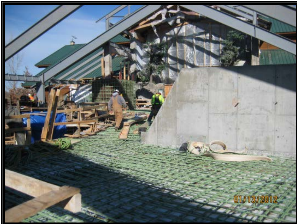
1316' Elevated Slab Rebar
