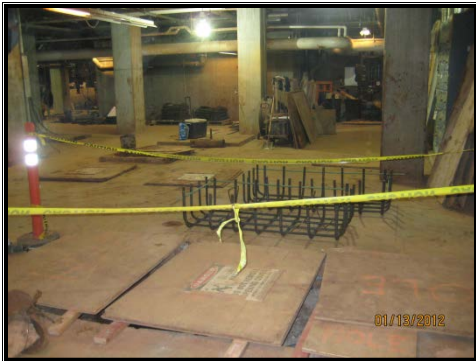
Basement Micro-Pile Installation
