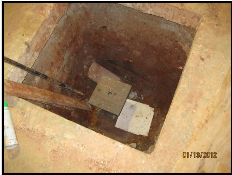
Basement Micro-Pile
