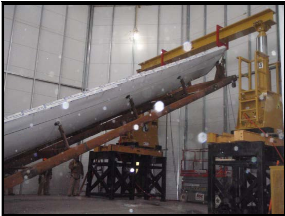
Lifting of Acrylic Panel with Gantry Crane
