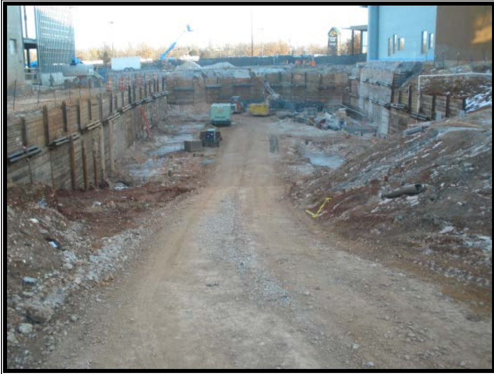
Snapshot of the Connector Excavation
