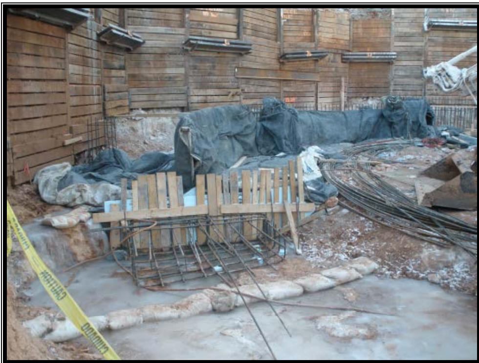
Installation of Concrete Footing
