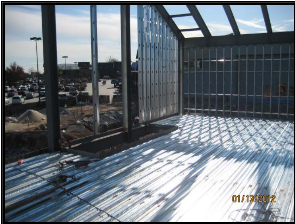
Back of House Structural Steel/Metal Deck
