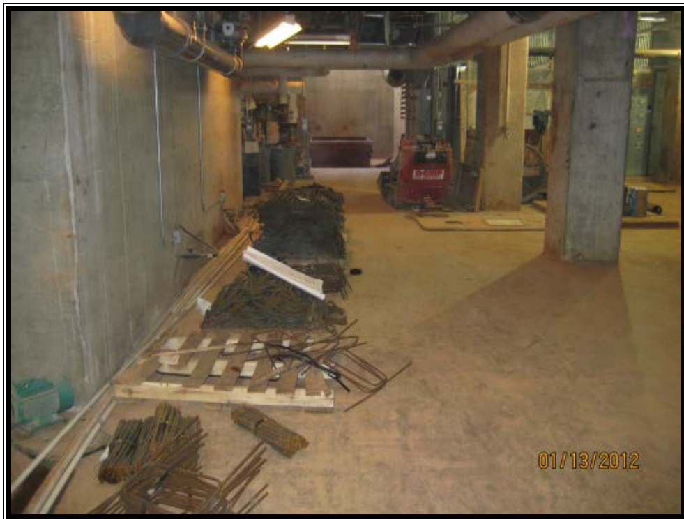
Basement Micro-Pile Rebar
