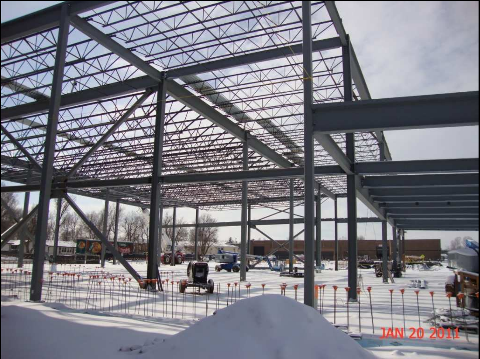
Steel Erection
