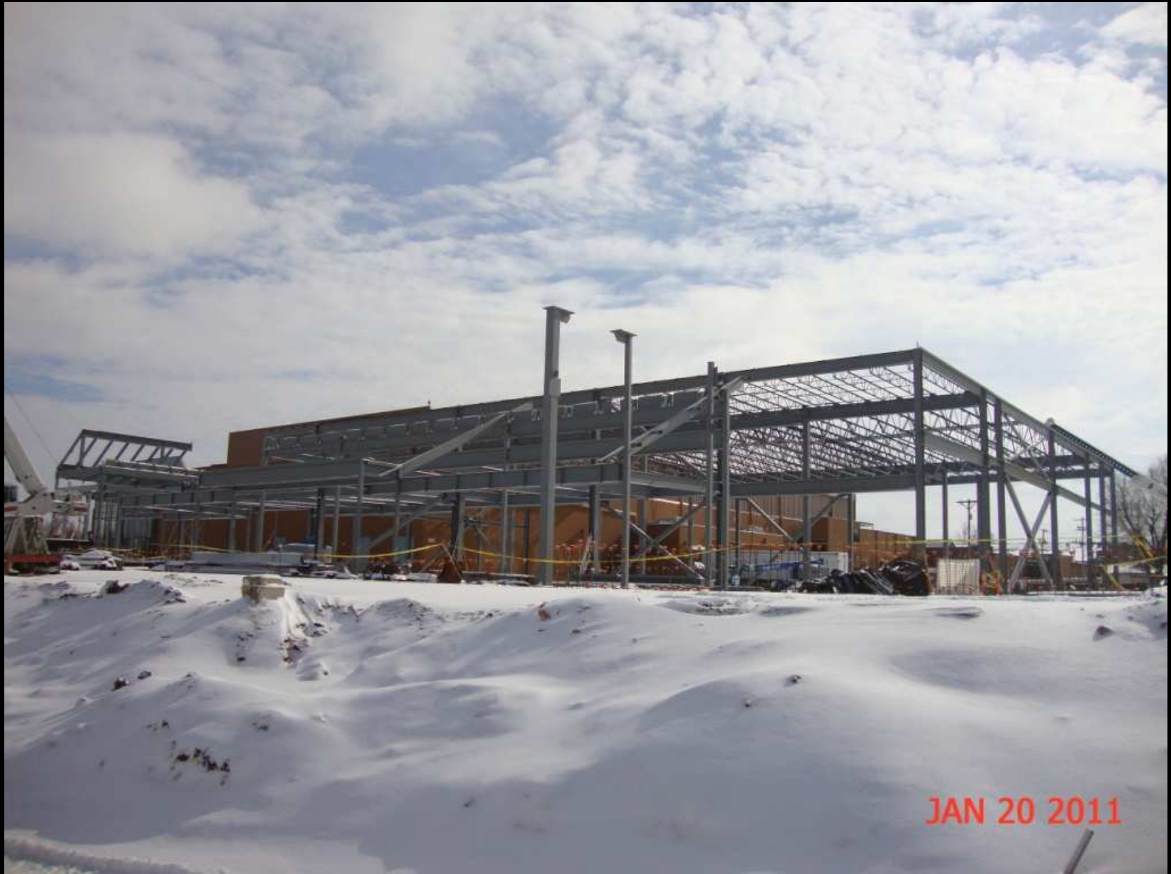
Steel Erection
