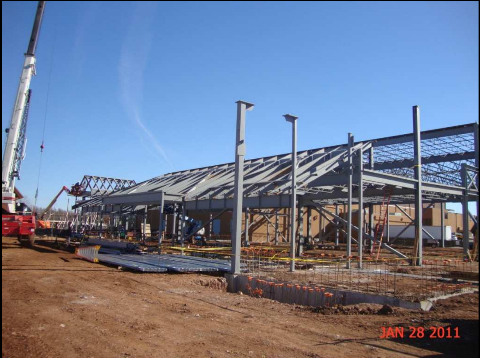
Steel Erection
