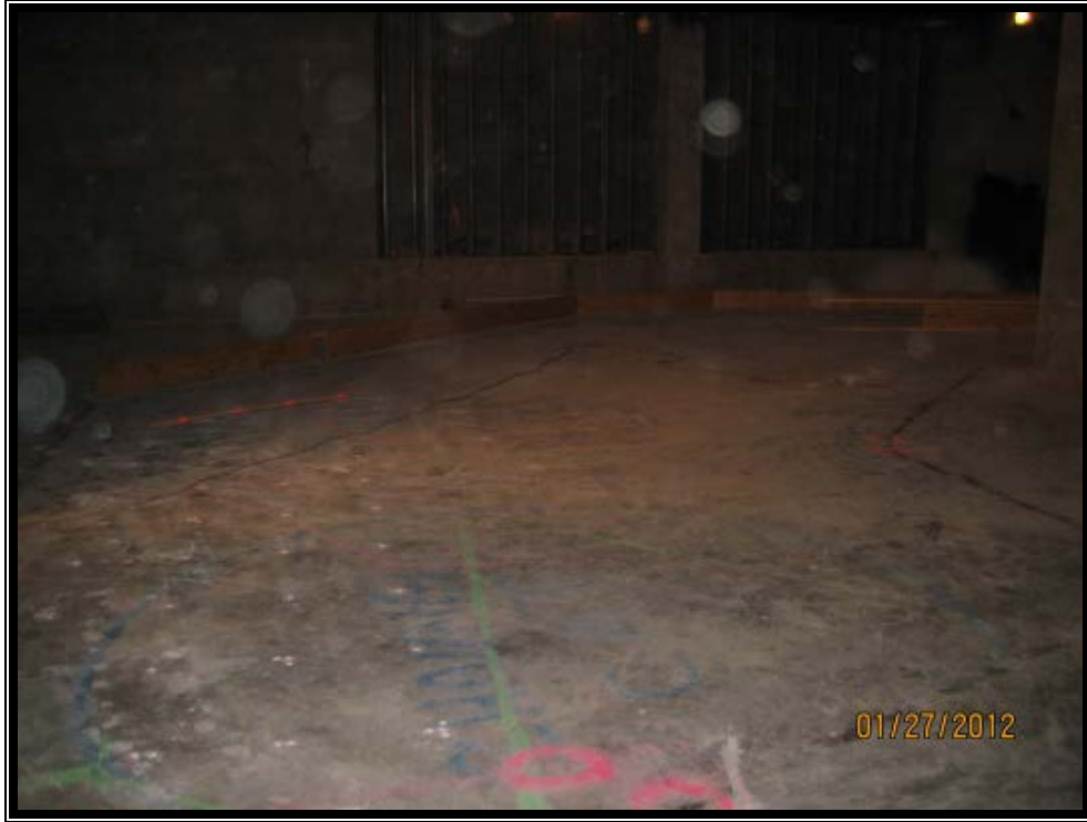
Under River Experience Concrete Forms
