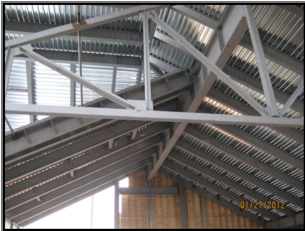
Back of House Structural Steel/ Roof Deck
