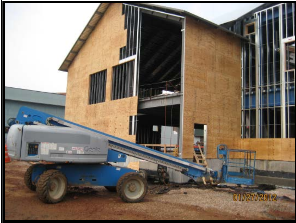
BOH Exterior Sheathing
