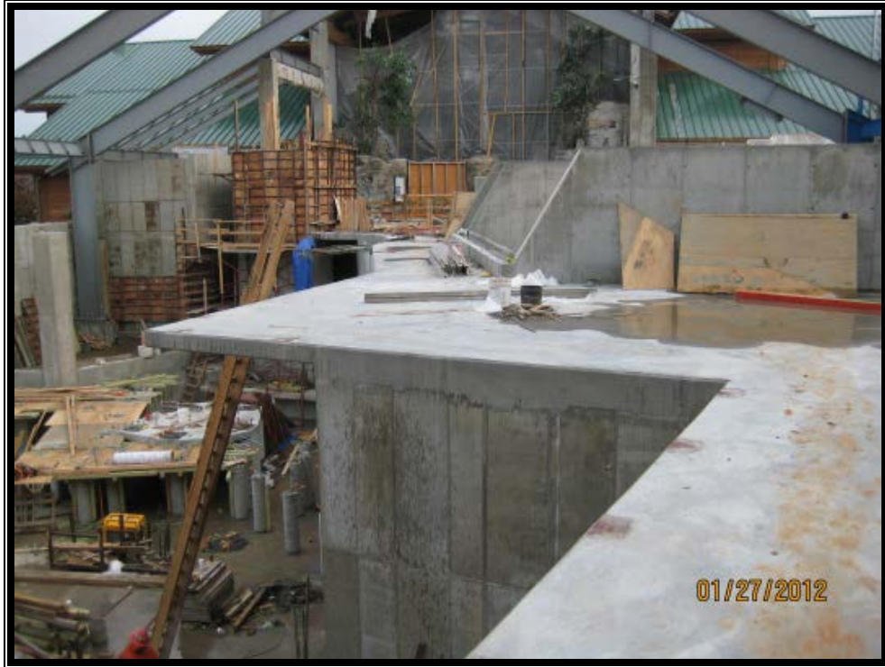
1316' Concrete Walkway Snapshot
