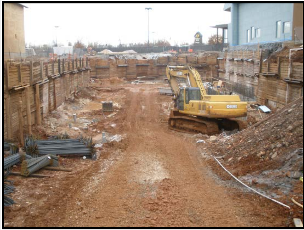
Snapshot of the Connector Excavation
