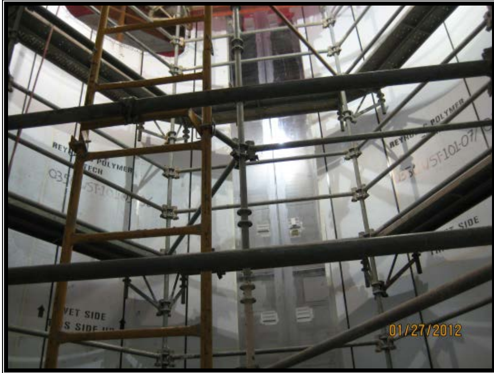
Scaffolding for Stingray Tank Acrylic Bonding
