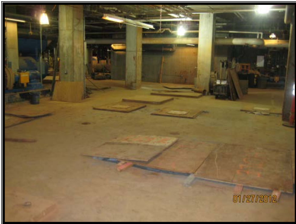
Basement Micro-Pile Snapshot
