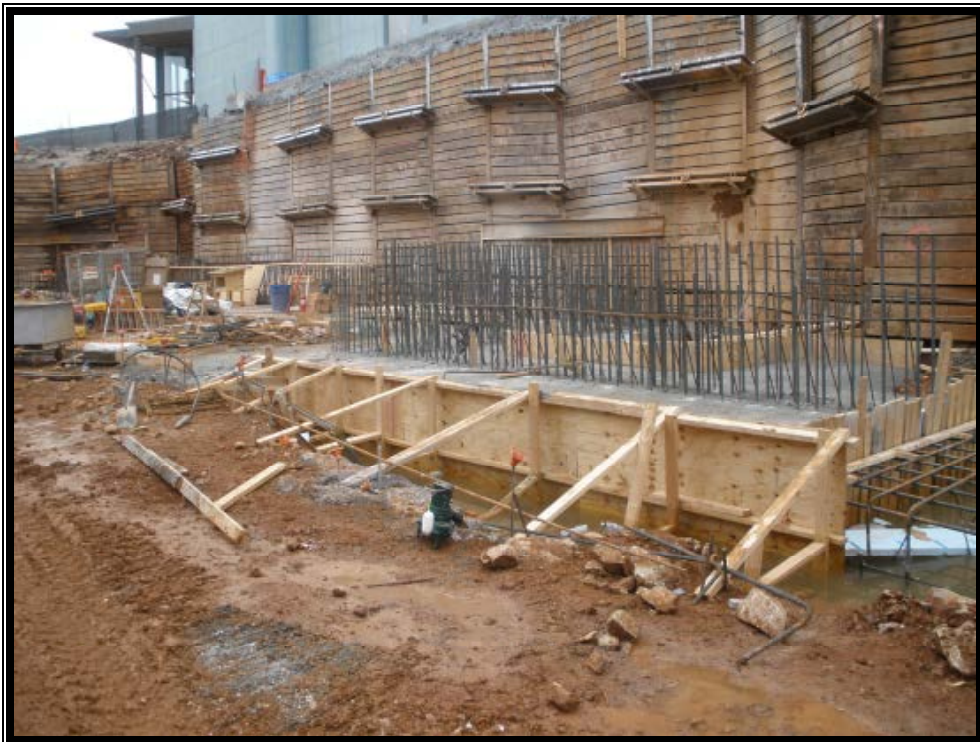
Installation of Concrete Footing
