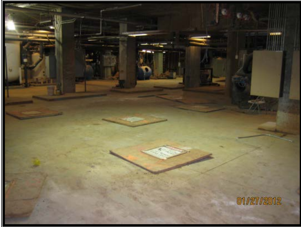
Basement Micro-Pile Snapshot
