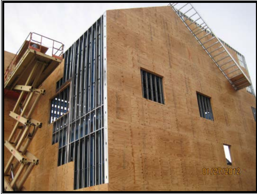
BOH Exterior Sheathing
