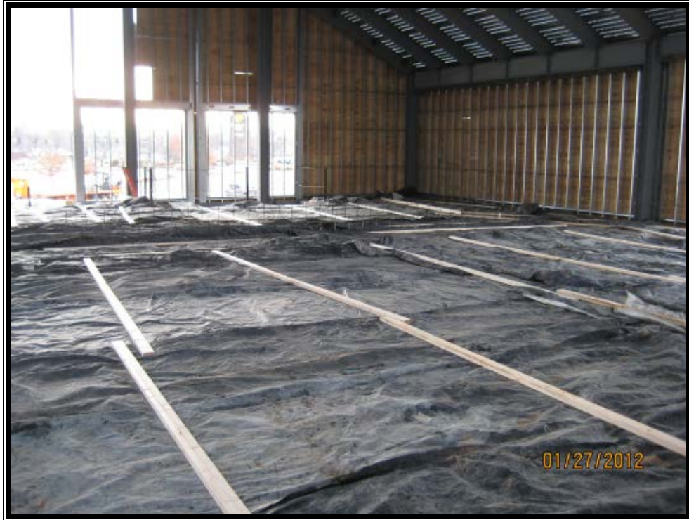
Metal Deck Concrete Slab
