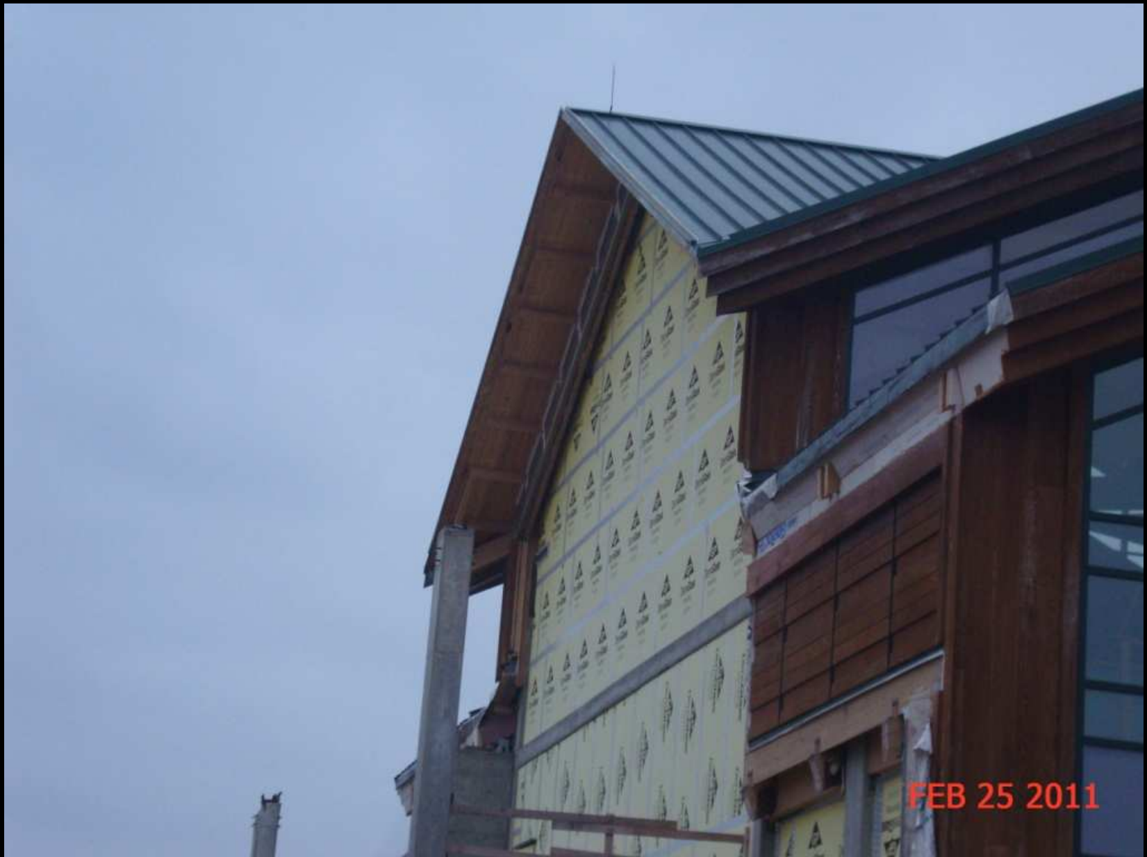
C Building Eave Demolition
