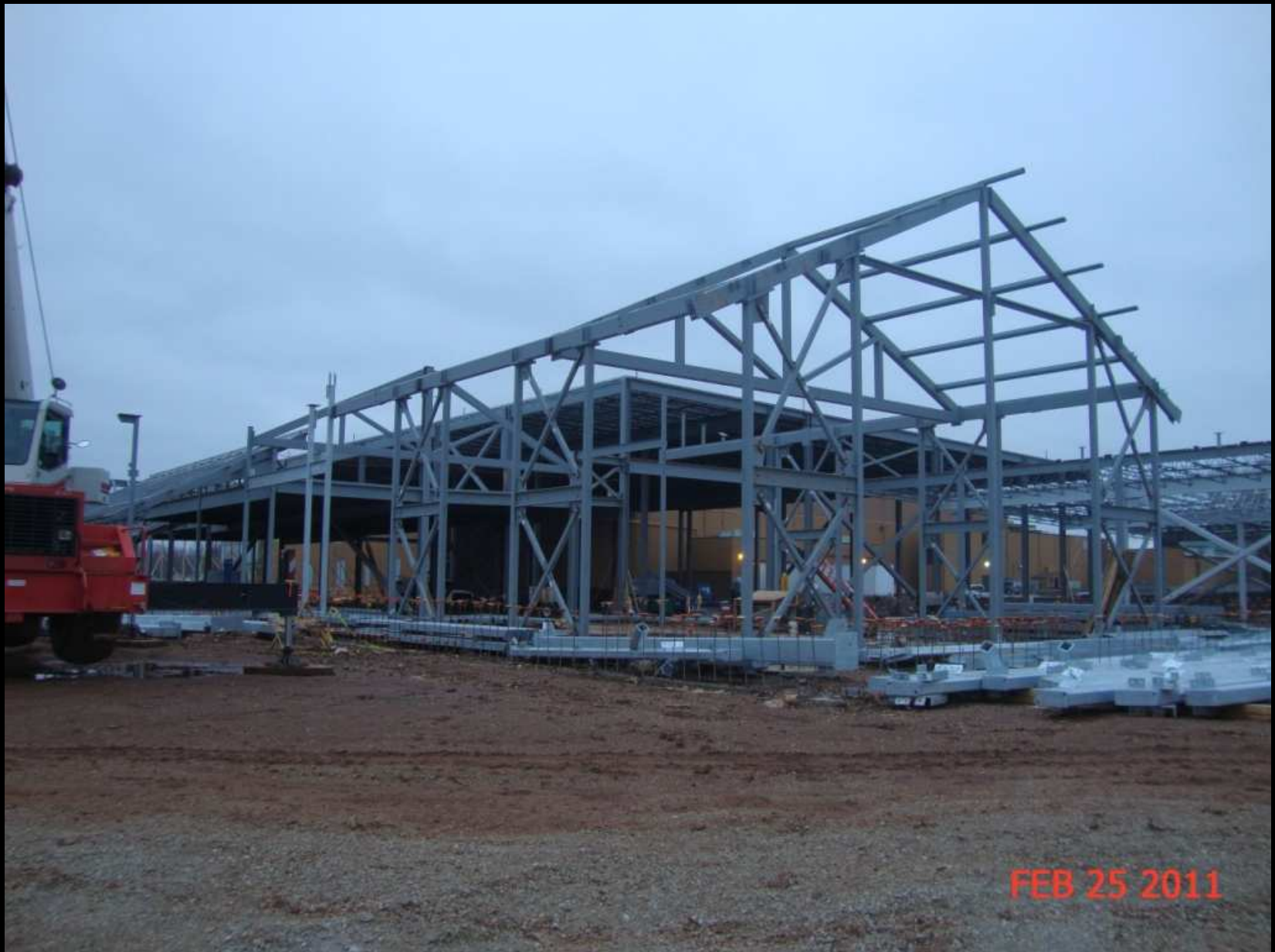
Sequence 4 Steel Erection
