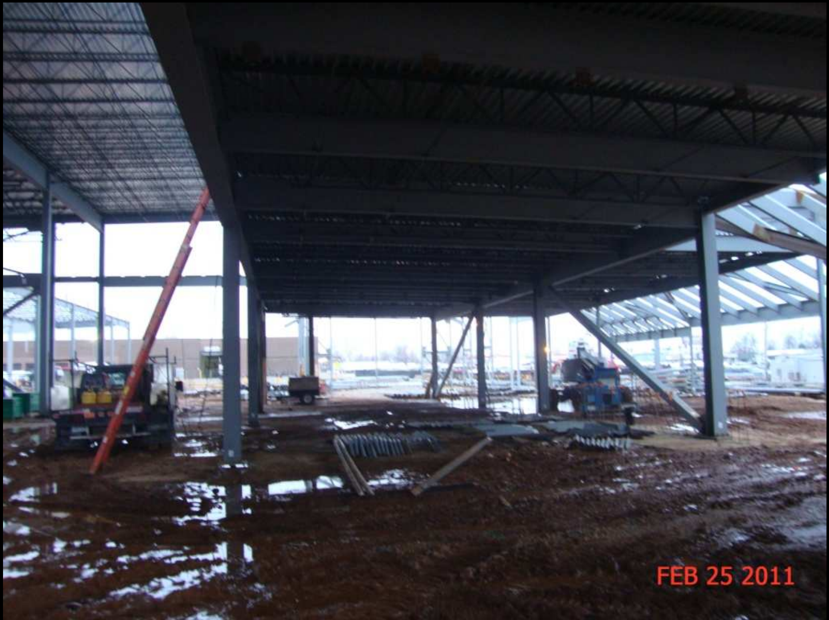
Sequence 3 Steel Detailing/Decking
