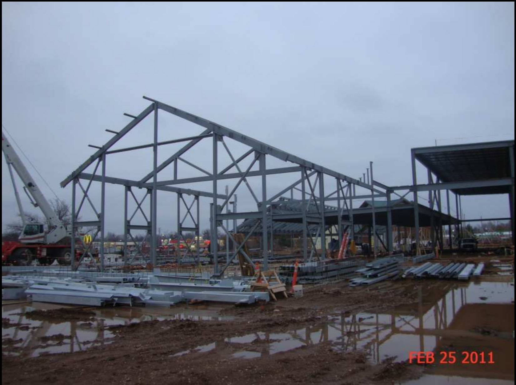
Sequence 4 Steel Erection
