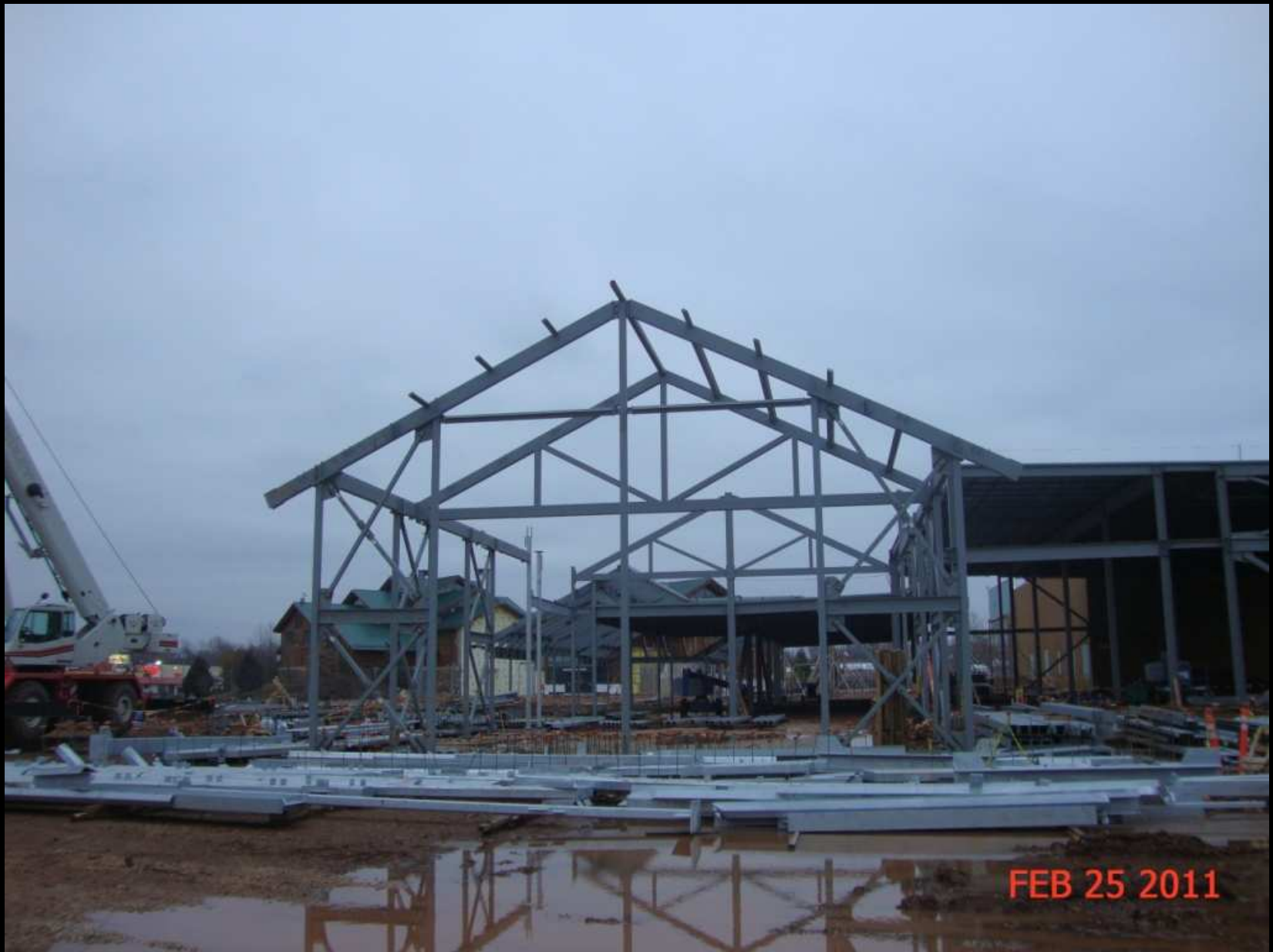
Sequence 4 Steel Erection
