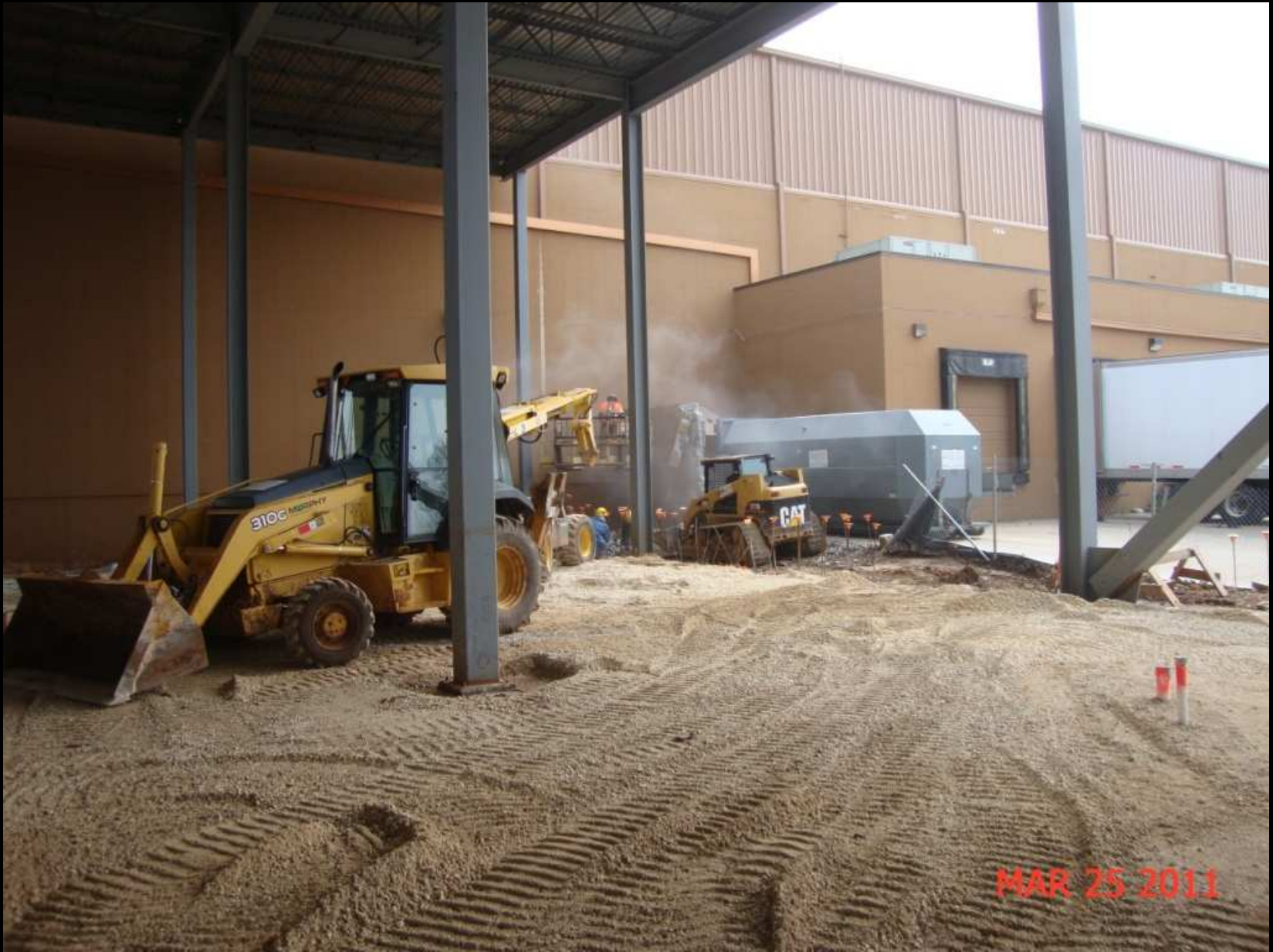
Demo of Screen Wall For Stairwell
