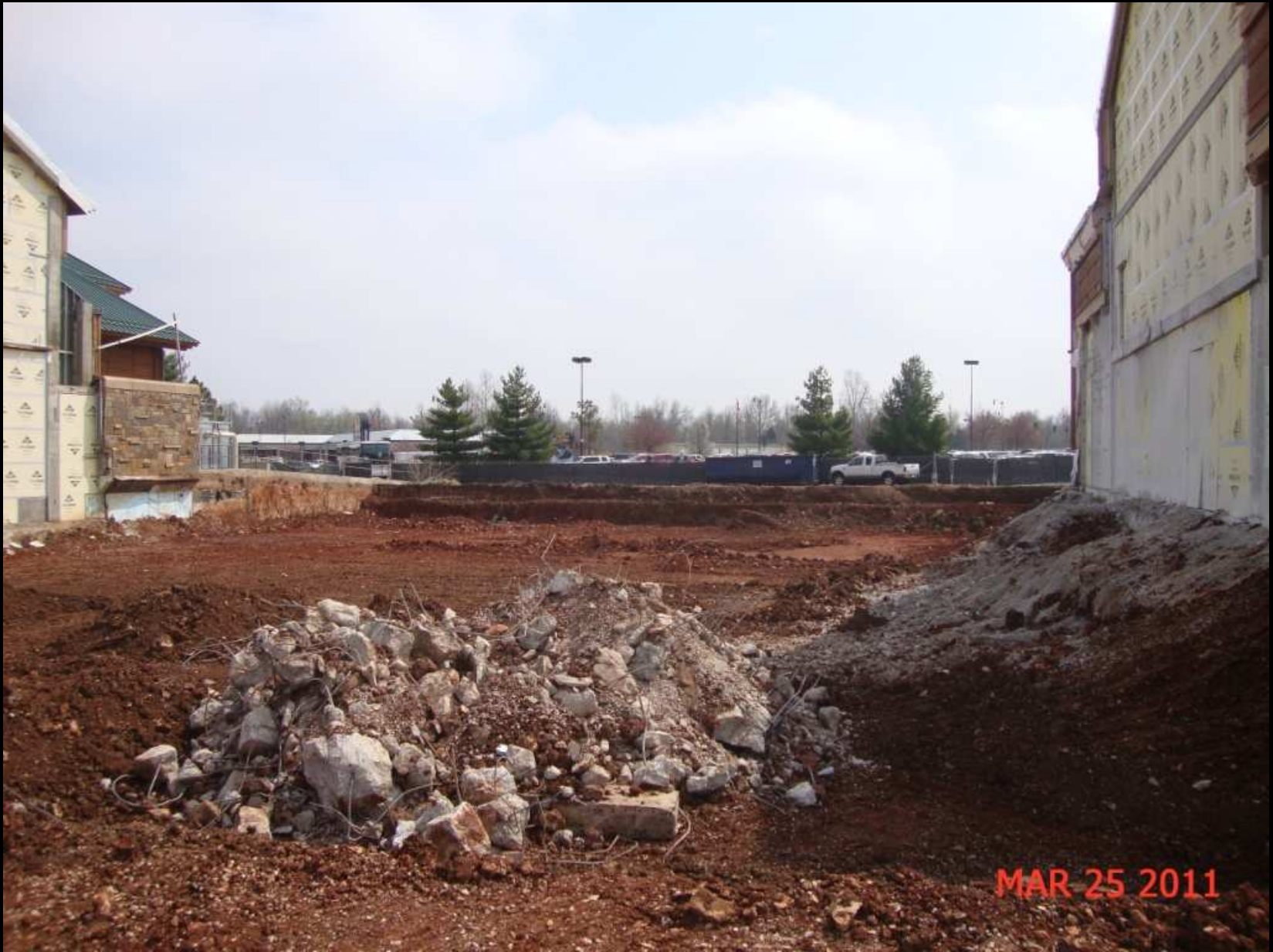
B Building Excavation
