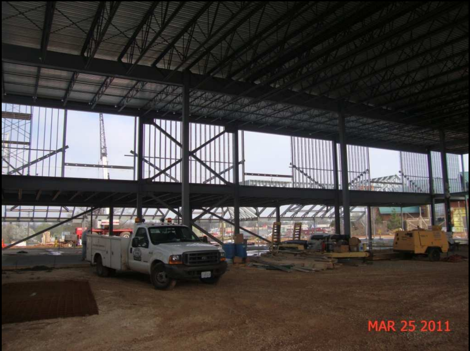
Framing Upper Roof
