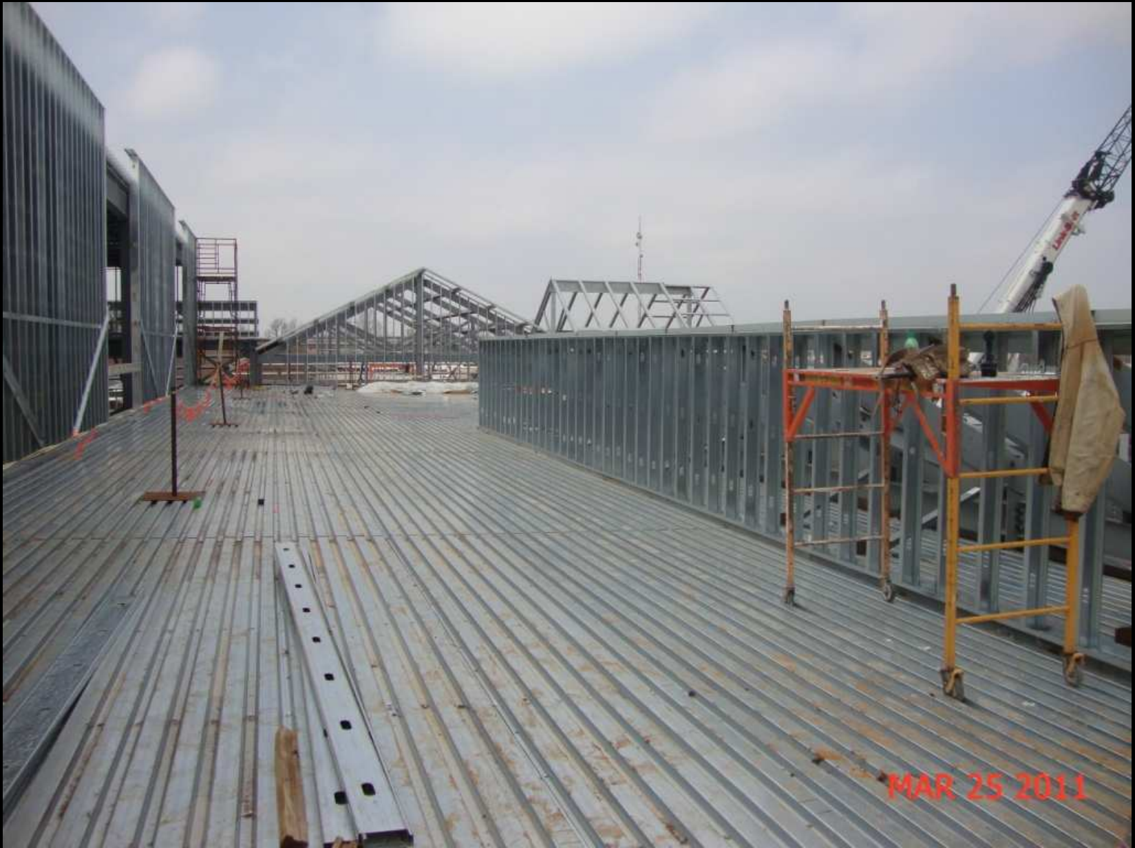
Framing Upper Roof
