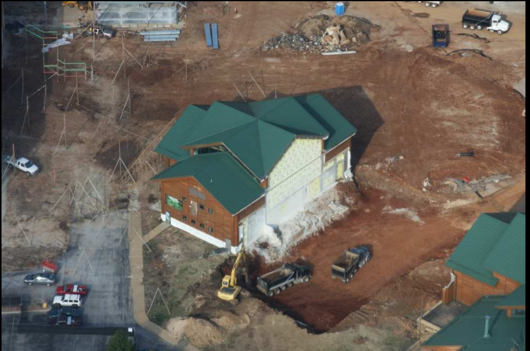
B Building Excavation
