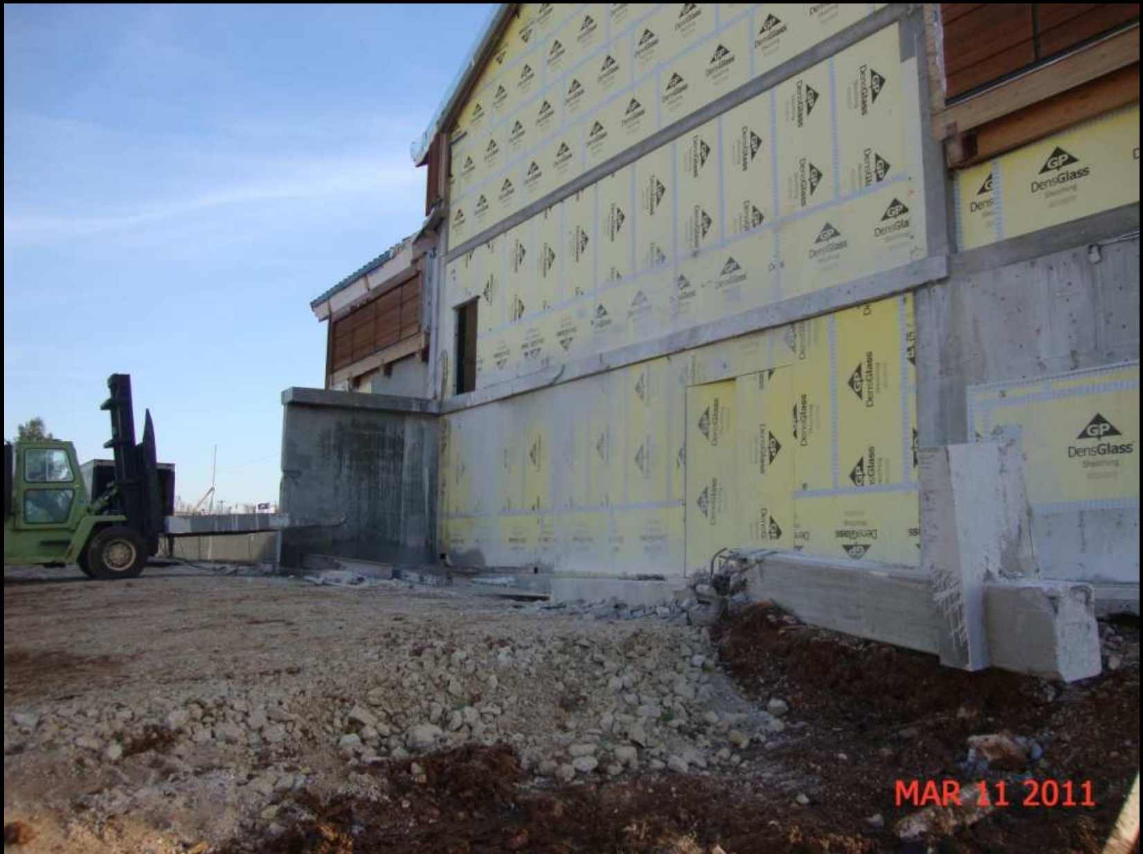
Demo C Building
