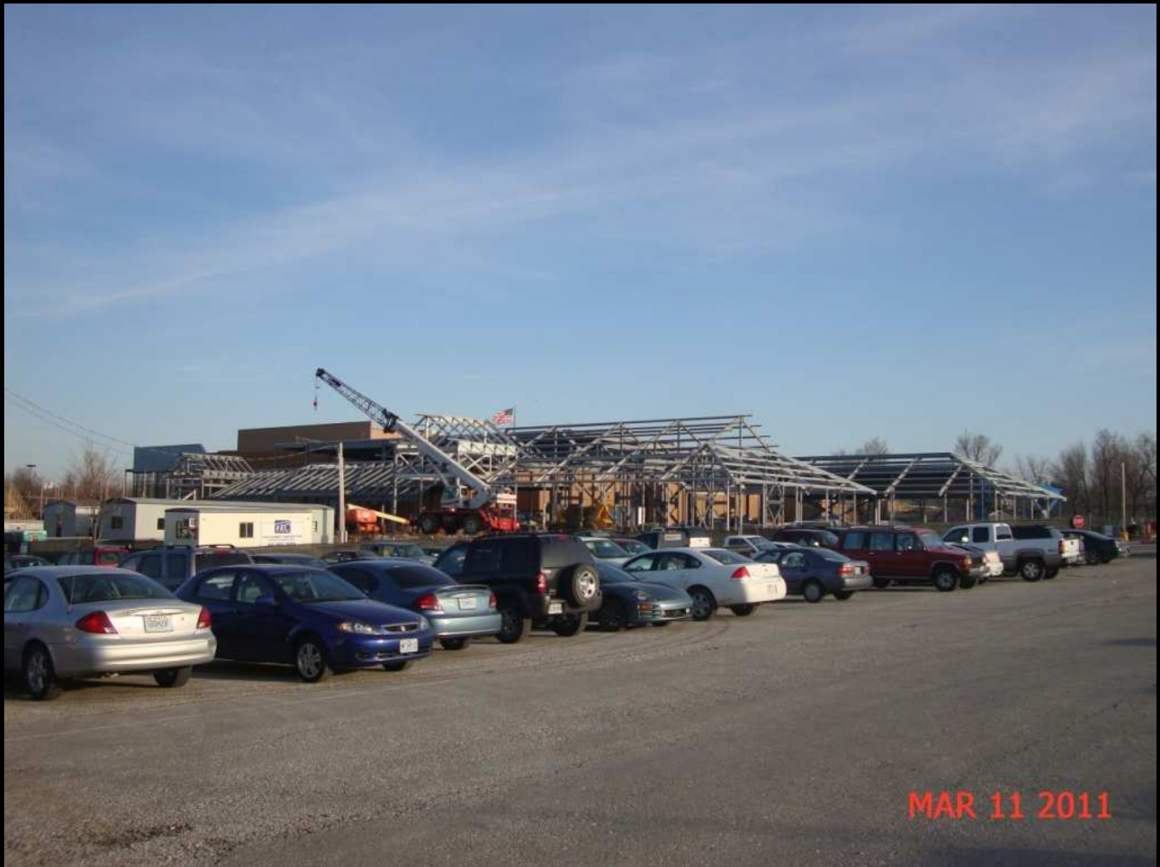
Steel Erection Overall View
