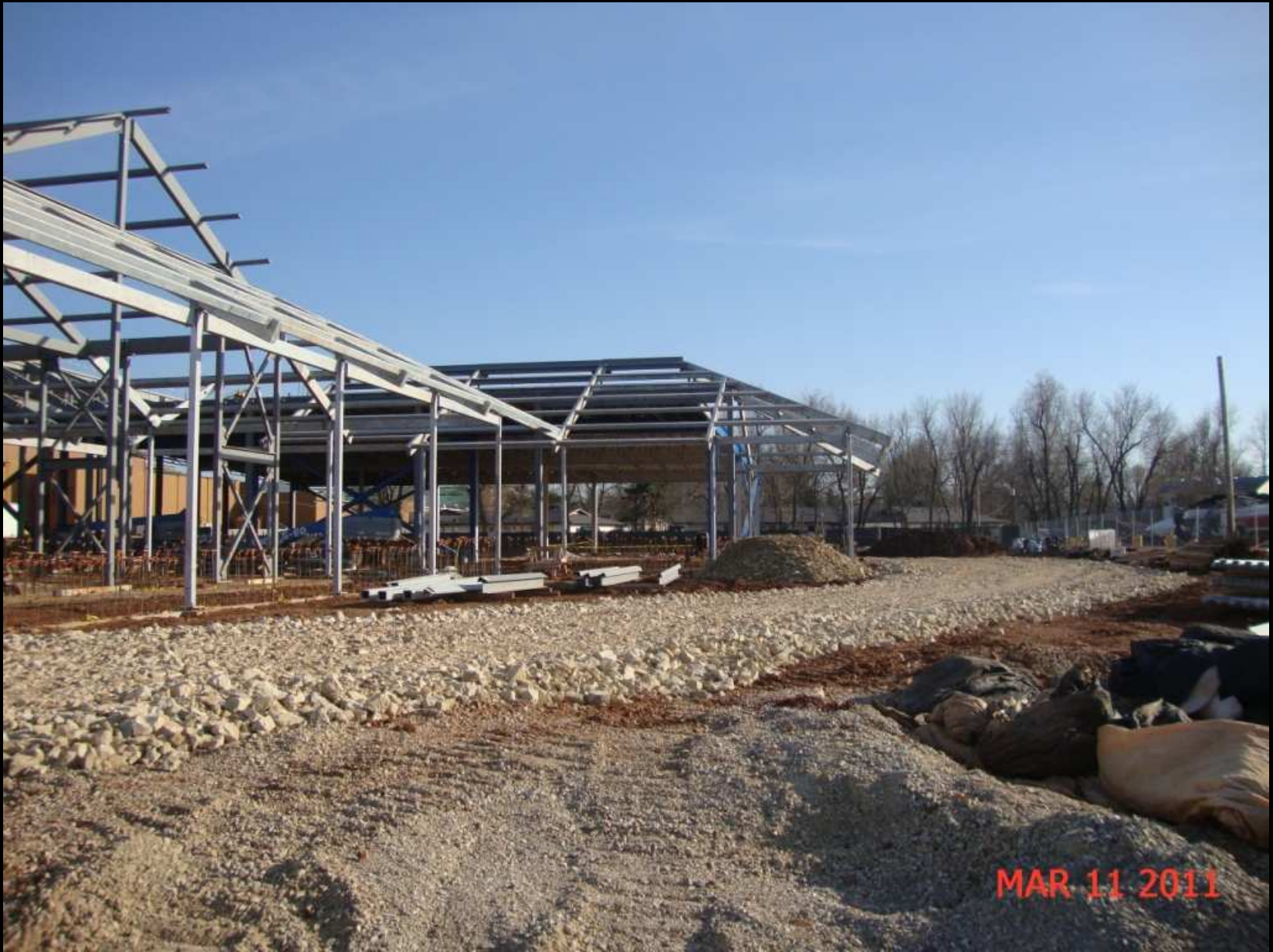
Steel Erection Sequence 4
