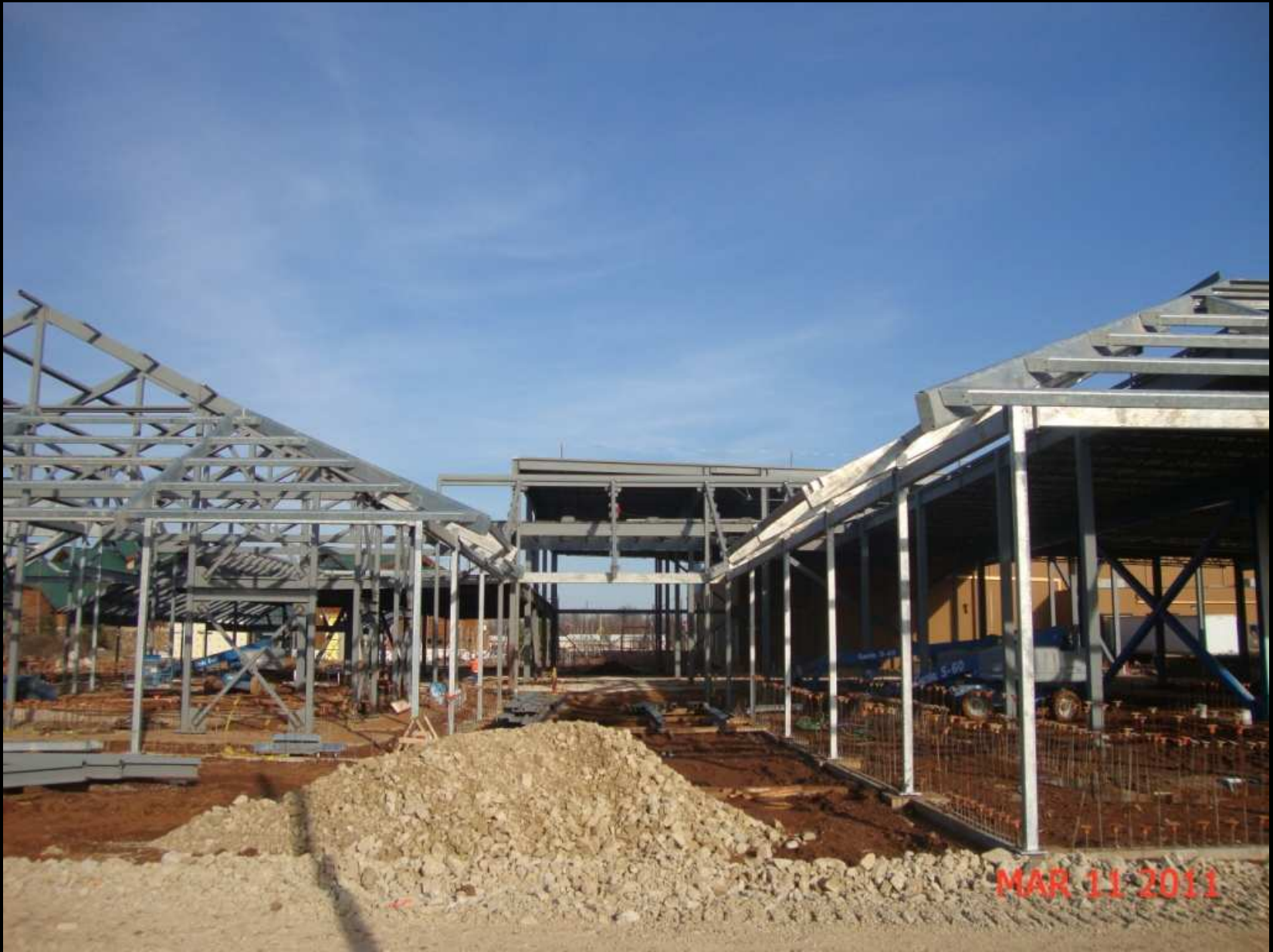
Steel Erection Sequence 4
