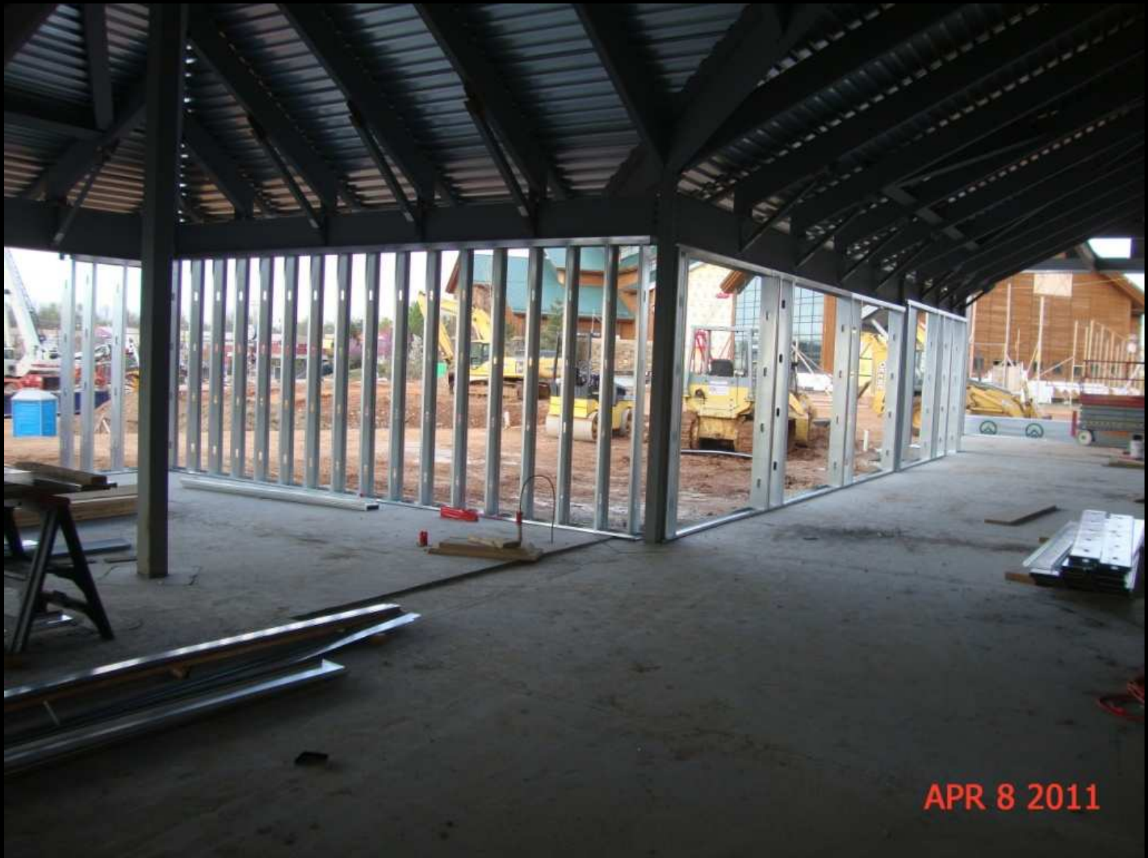
Exterior Wall Framing
