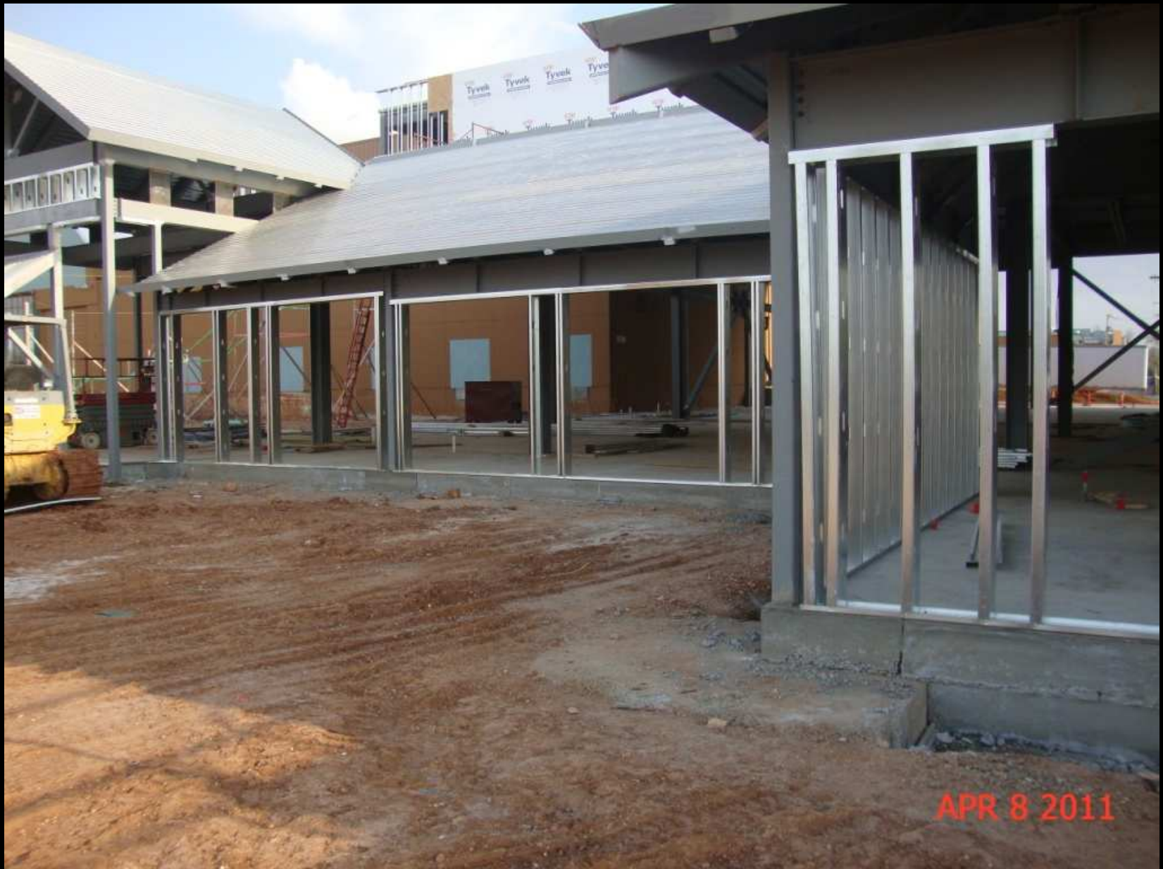
Exterior Wall Framing
