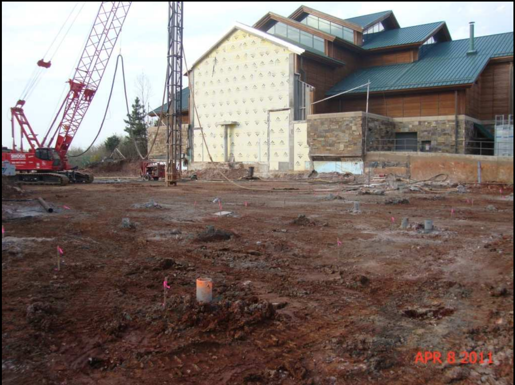
Macro Pile Installation
