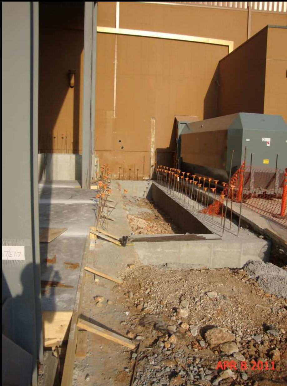
Foundations Stairwell
