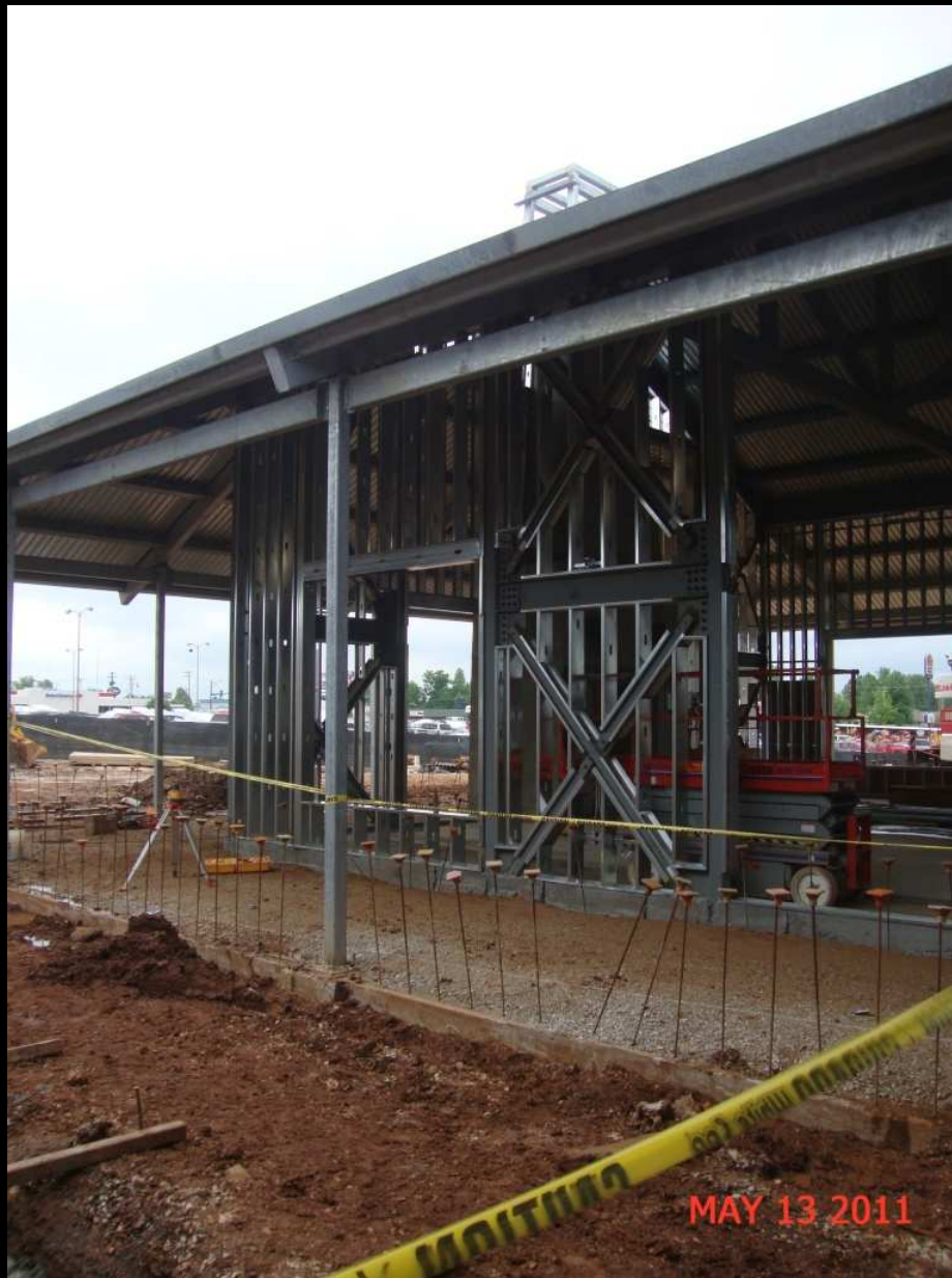
EXTERIOR FRAMING/SHEATHING
