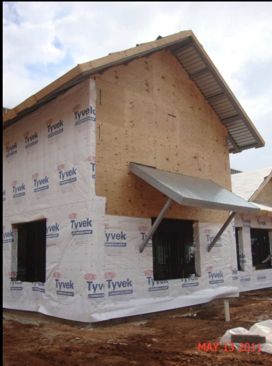
EXTERIOR FRAMING/SHEATHING
