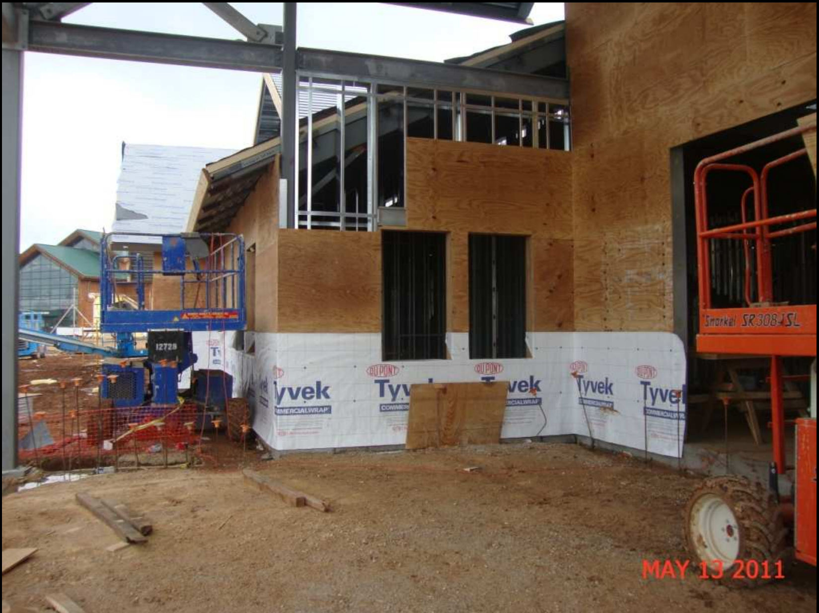
EXTERIOR FRAMING/SHEATHING
