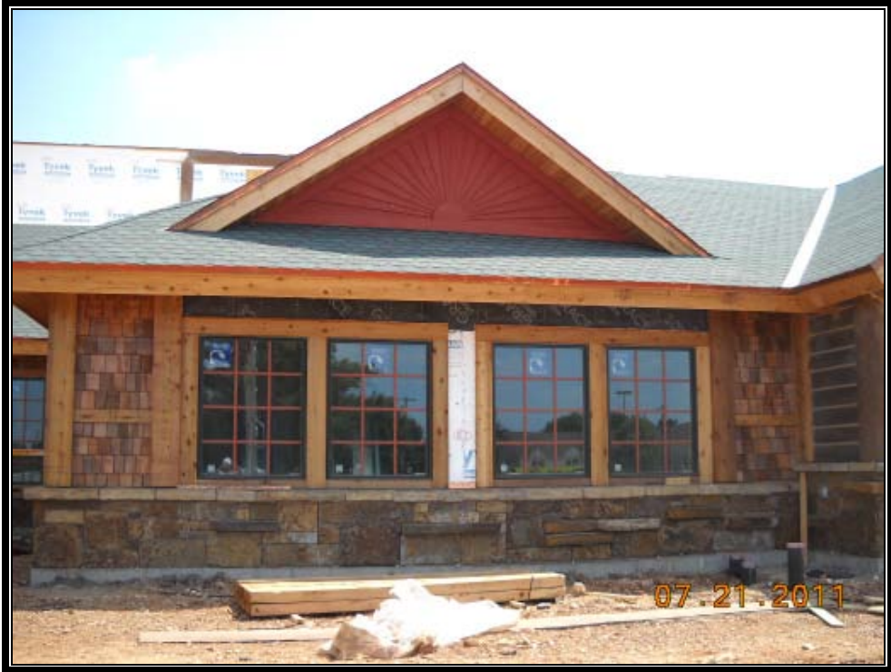
Cajun Red Paint Mock-up & Installation of Cedar Shakes and Exterior Trim
