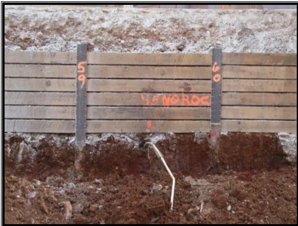
Tie-back with Tensioning Cables Installed
