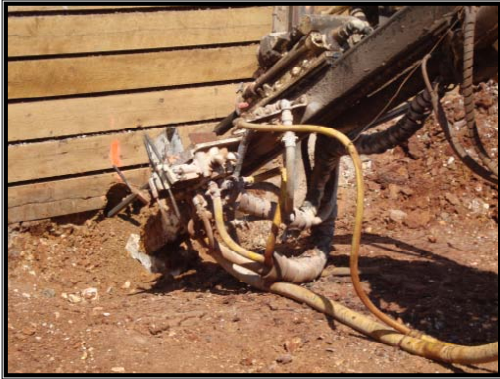
Drilling for Tie-backs
