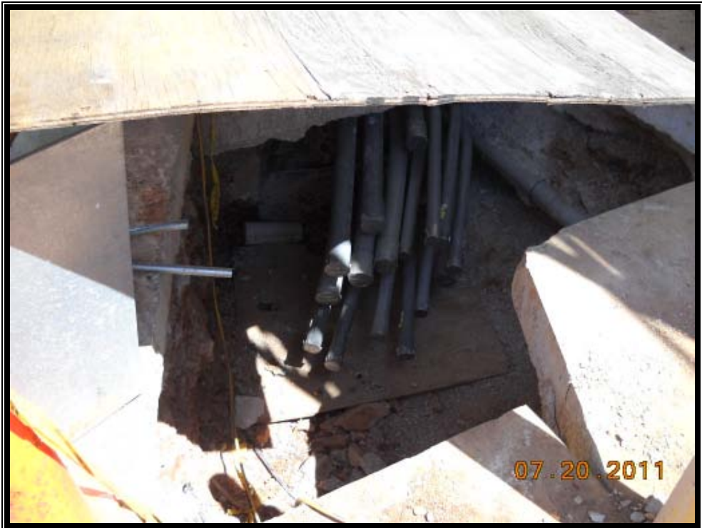
Underground Electrical Duct Bank Tie-In
