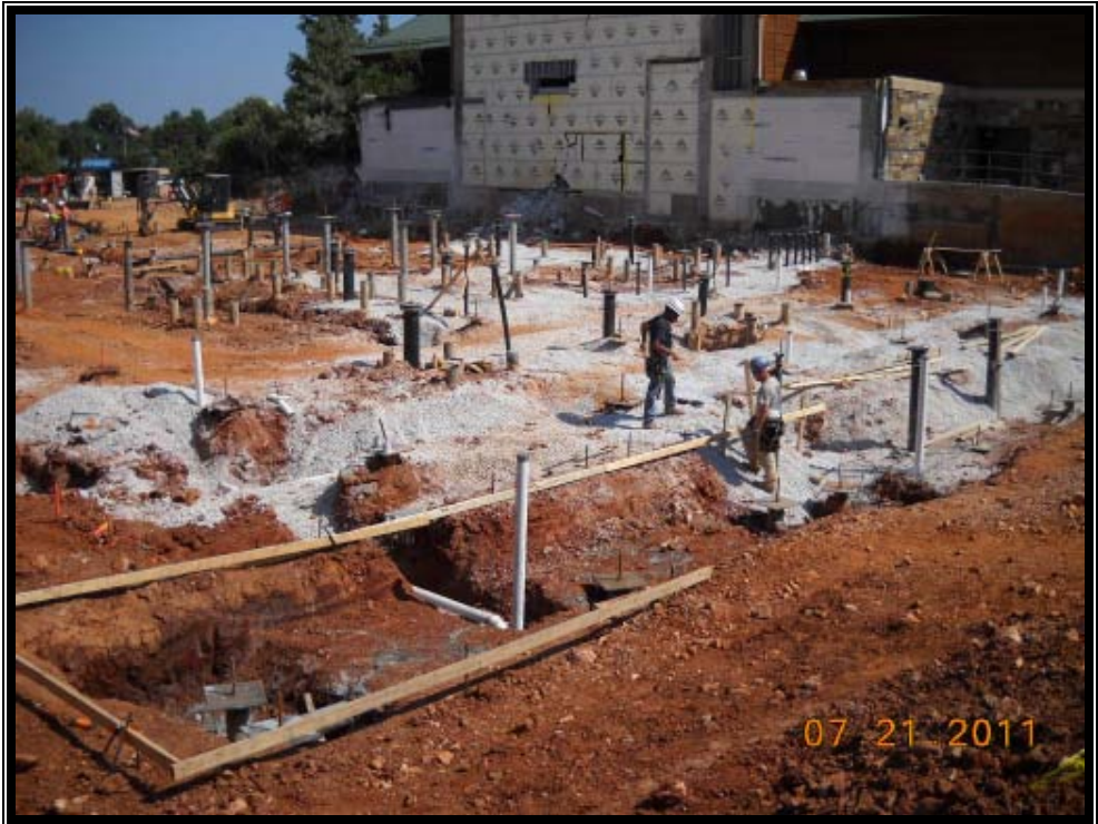
Footing Formwork and Preparation
