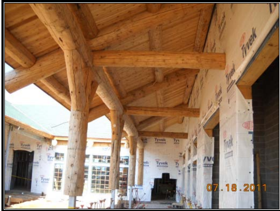
Installation of Exterior Decorative Timbers Outside of Lab E163
