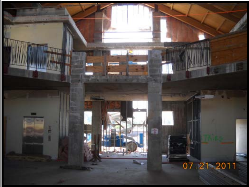
Exterior Skin and Metal Stud Demolition
