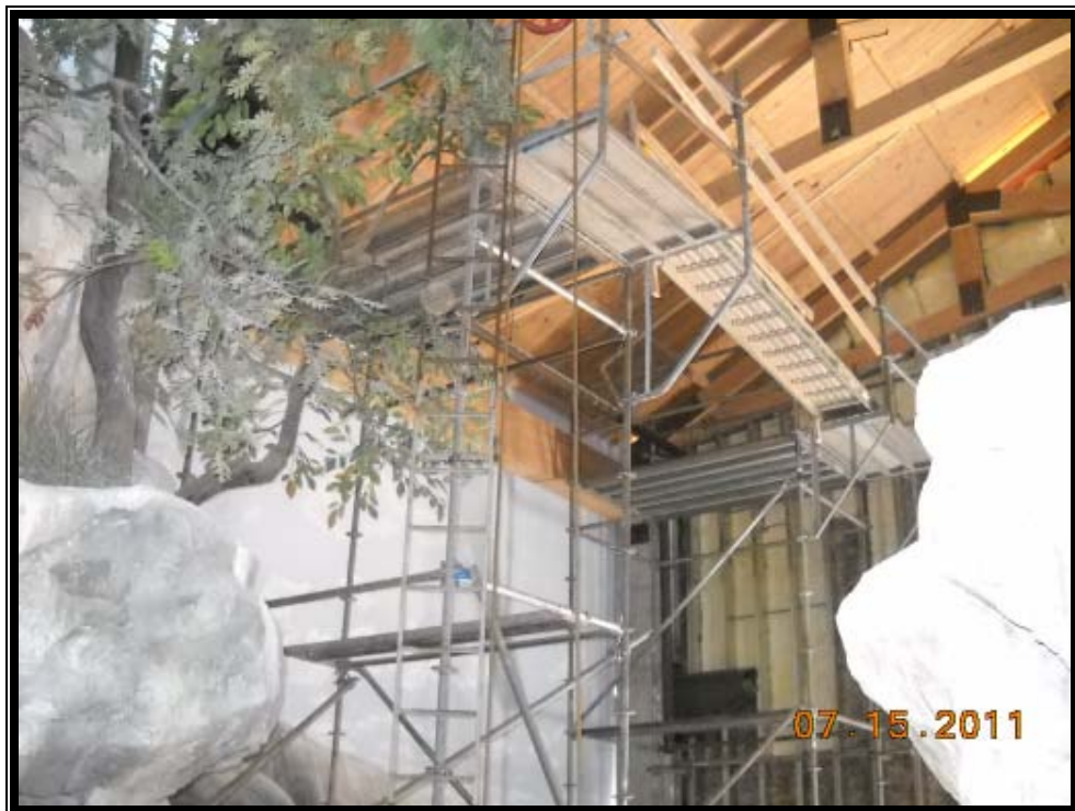
Scaffold Towers for Overhead Light Removal
