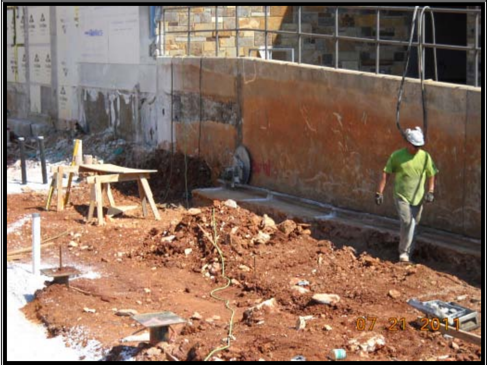
Existing Footing Removal
