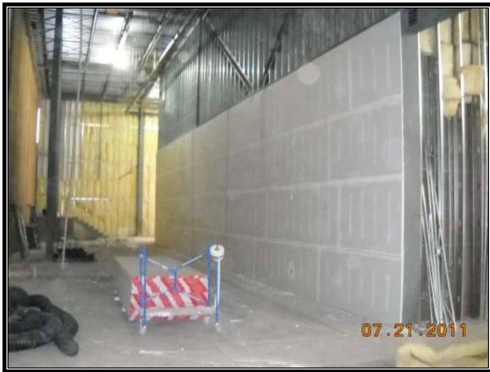
Installation of Drywall Corridor E120 and Warming Kitchen E123
