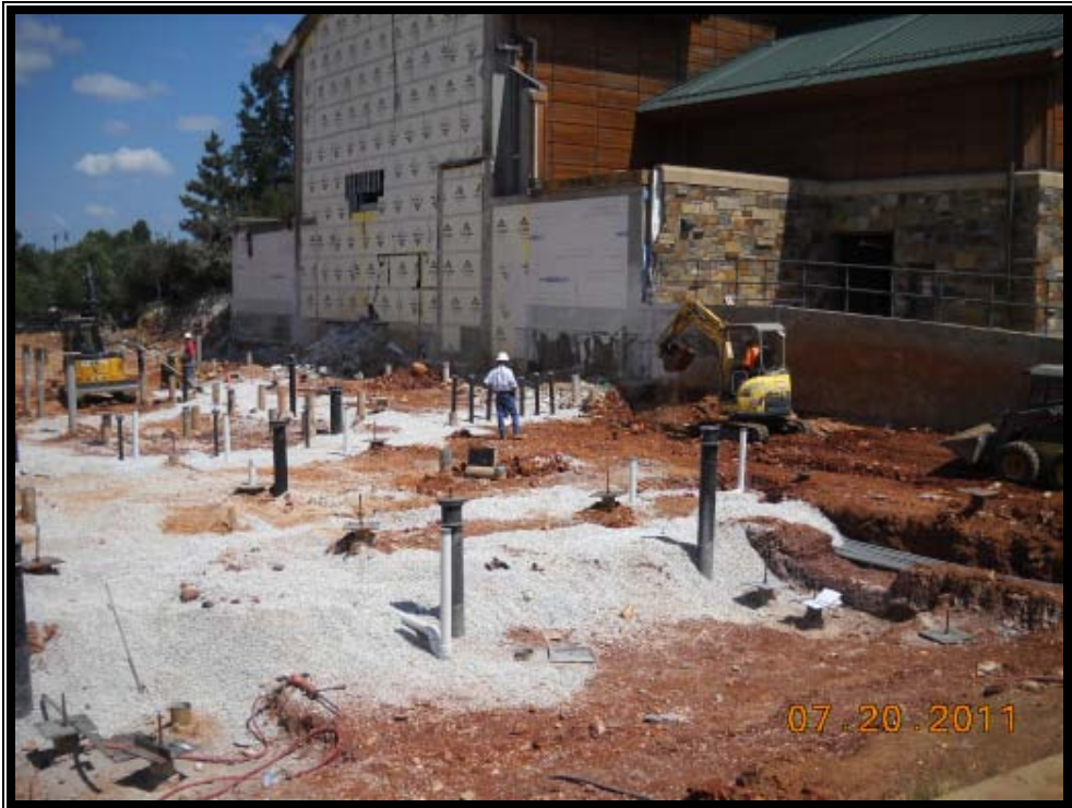
Underground Polyethylene Pipe
