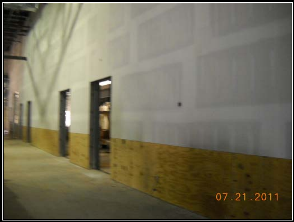
Drywall and Plywood Sheathing on North Expo Hall Wall
