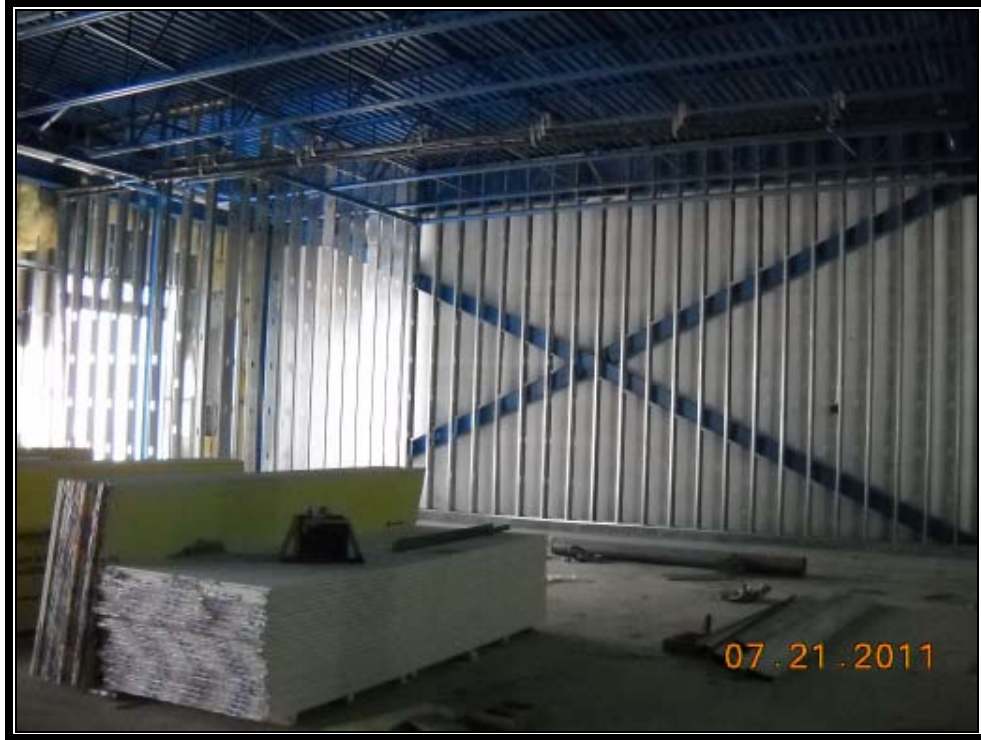
Installation of Drywall and Metal Framing in Southwest Corner of E153
