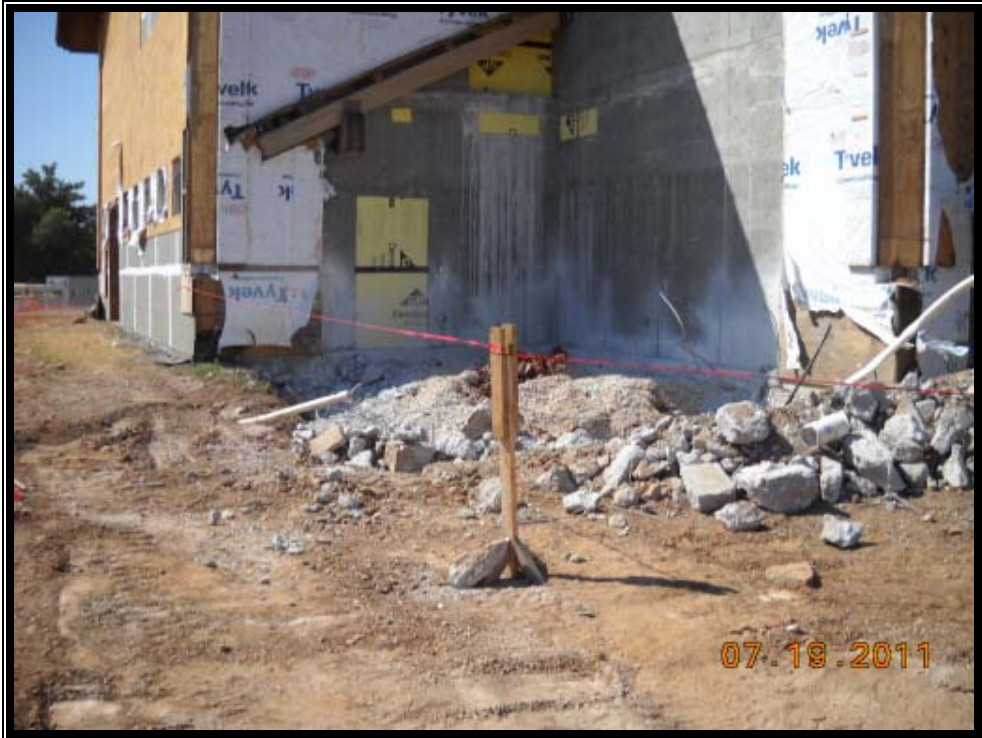
Slab on Grade and Footing Demolition
