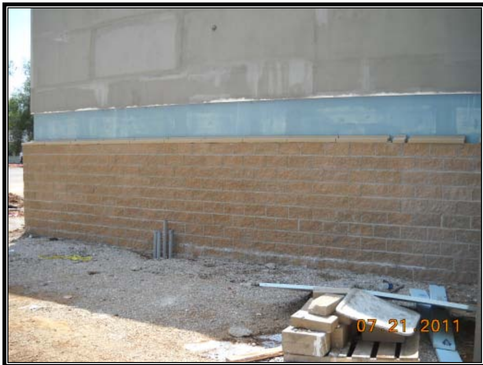
Installation of EIFS and CMU Wall with Cap
