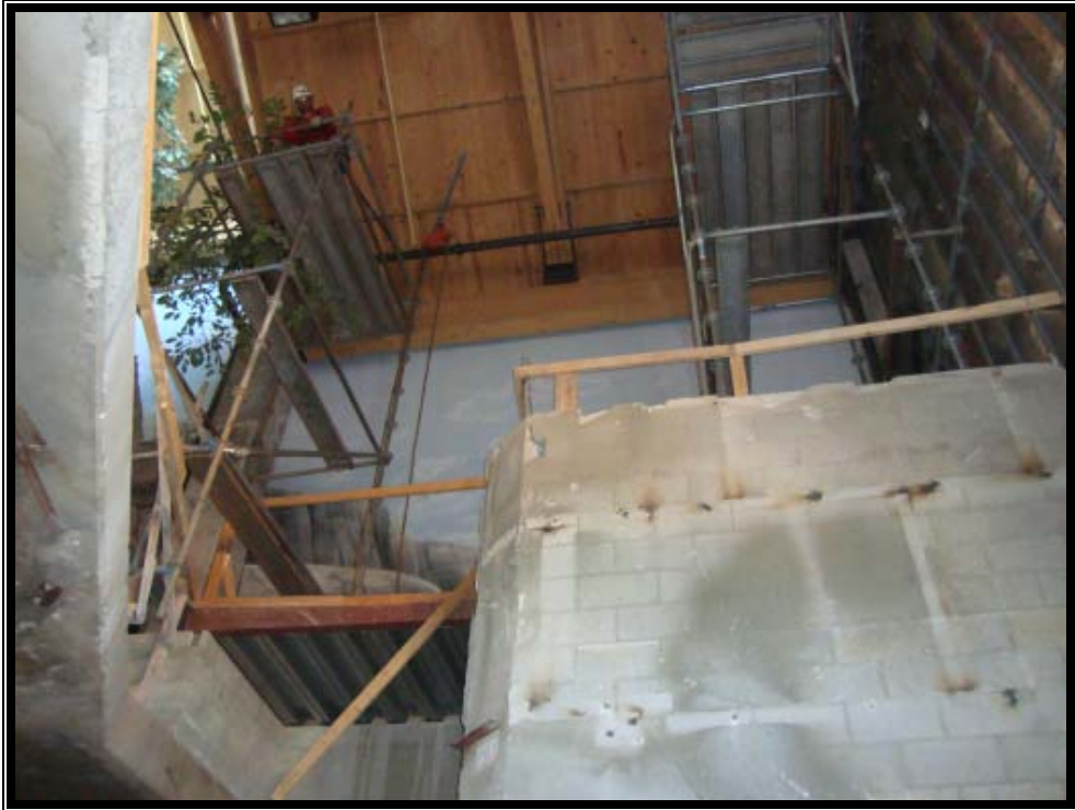
Scaffold Towers for Overhead Light Removal
