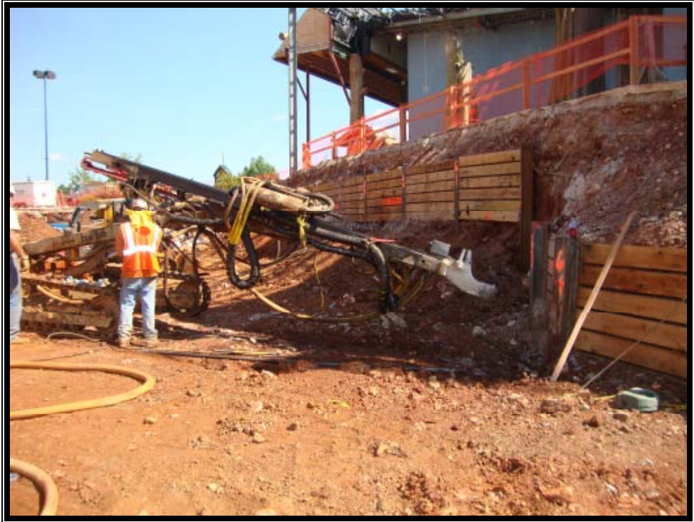
Drilling Tie-backs
