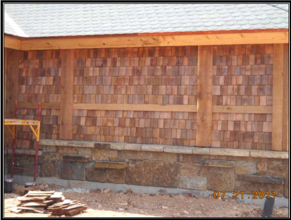
Installation of Cedar Shakes and Exterior Wood Trim
