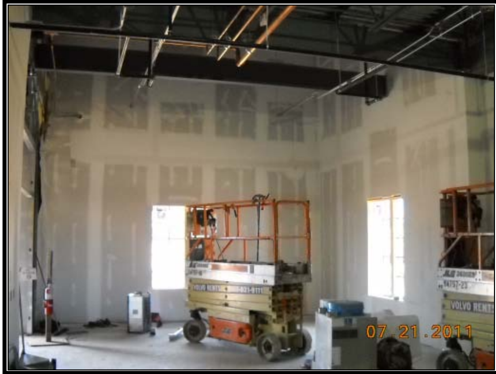
Installation of Drywall in CEC Lunchroom E117
