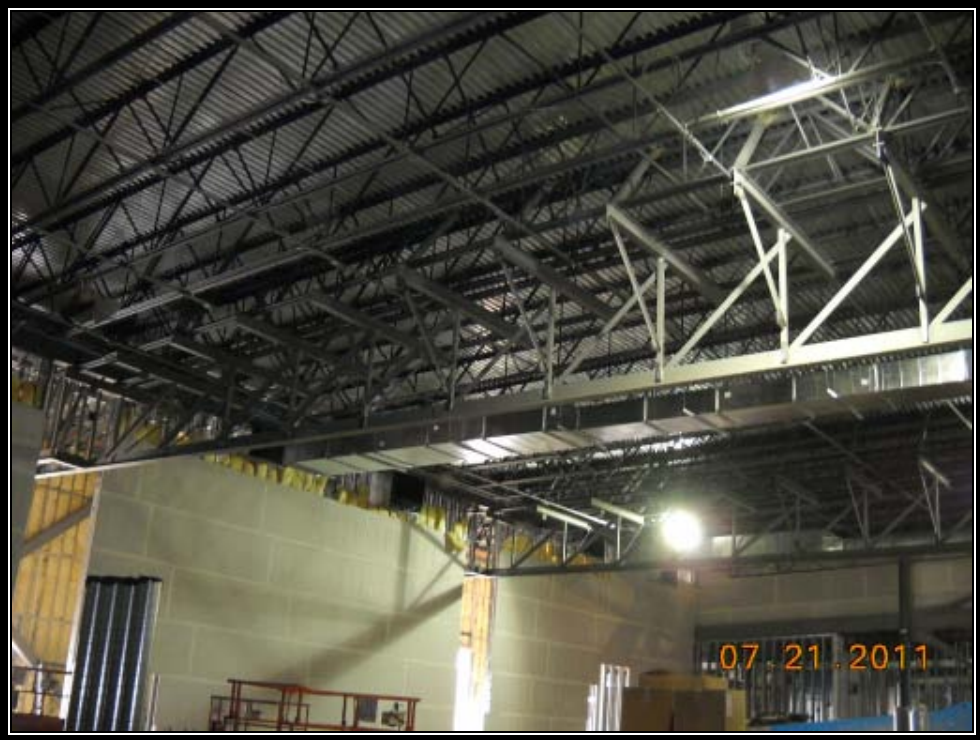
Installation of Operable Partition in Expo Halls E133, E134, and E135
