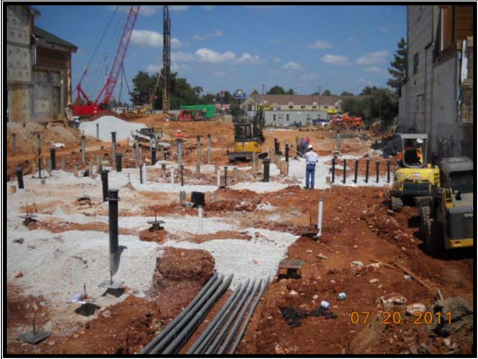
LSS Pipe Installation
