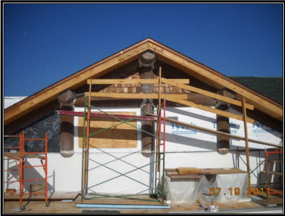
Installation of Cedar Shakes and Fiberglass Log
