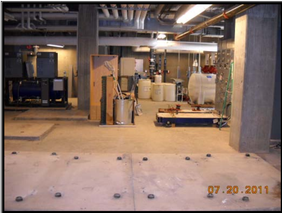
Shock Absorber Pad Removal Completion
