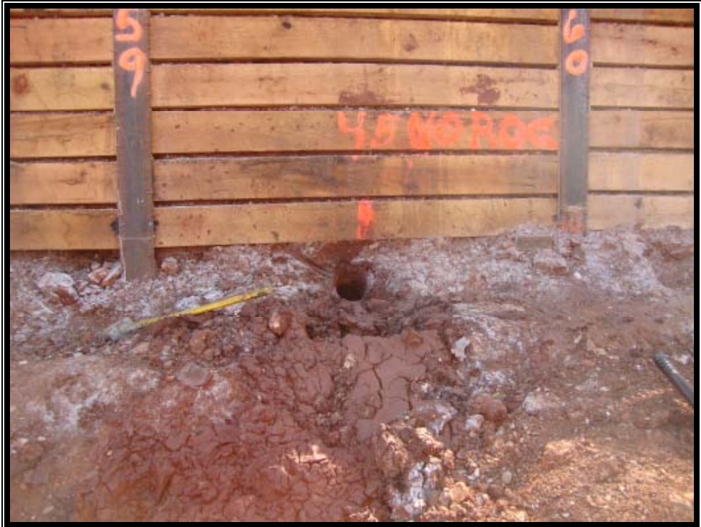
Tie-back Prepared for Grout
