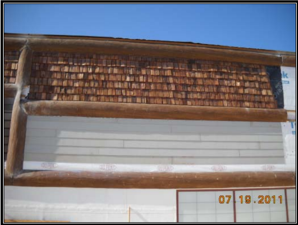
Installation of Cedar Shakes and Fiberglass Logs
