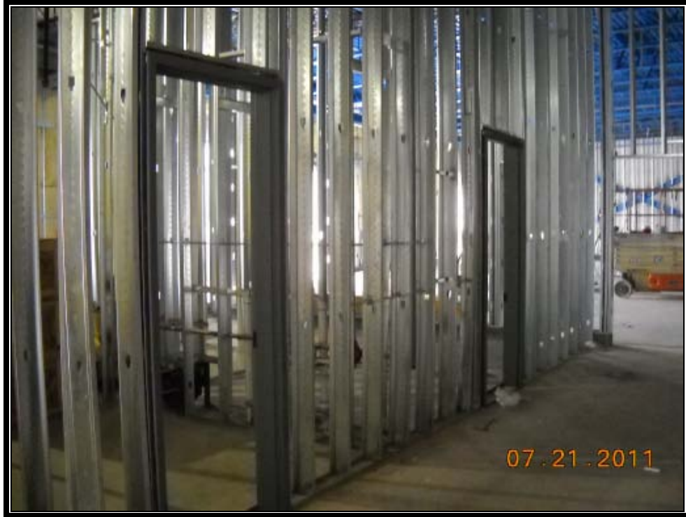
Installation of Door Frames
