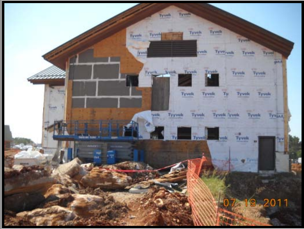
East-Exterior Skin Removal
